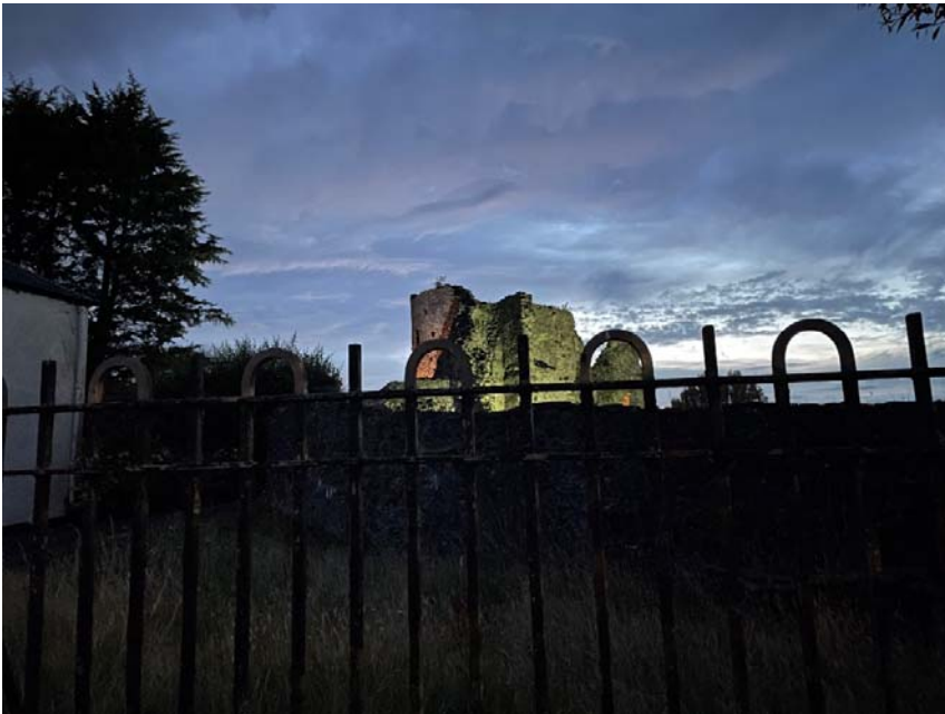
Plate 2 Castle lighting alongside northern elevation
