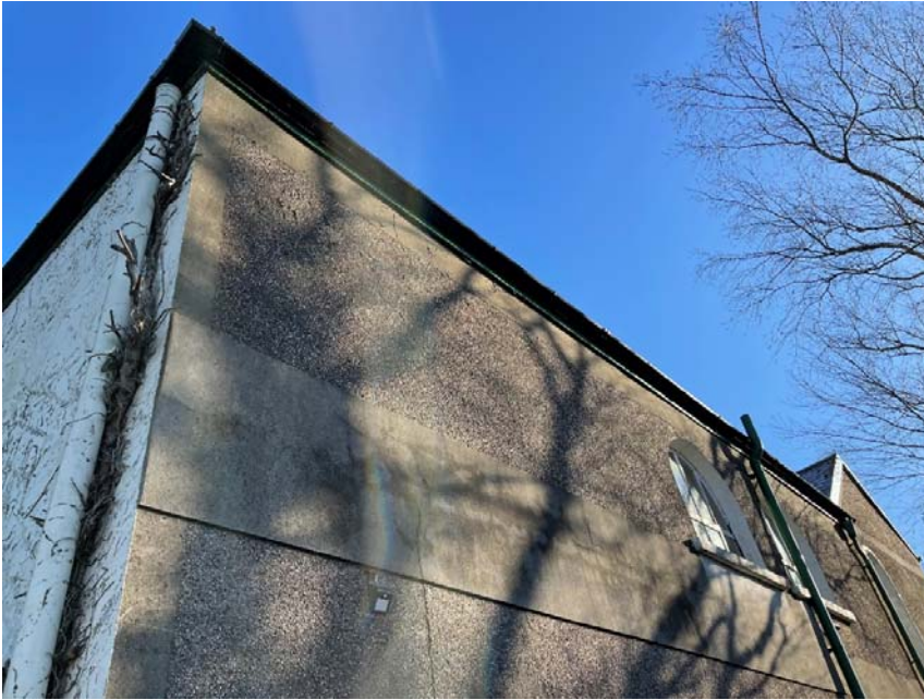
Plate 1 Surveyor view on western elevation. Photo taken during January day-time inspection
