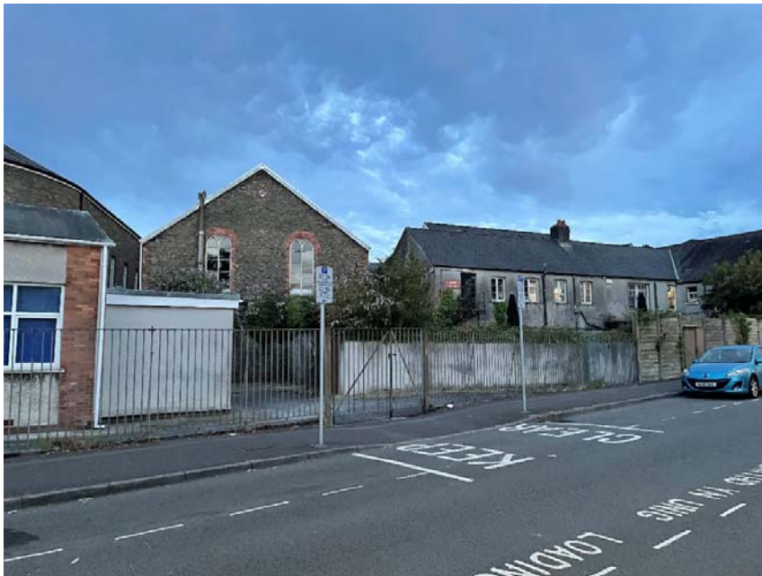
Plate 3 Rear of Buildings south of Castle Street where regular bat activity recorded
