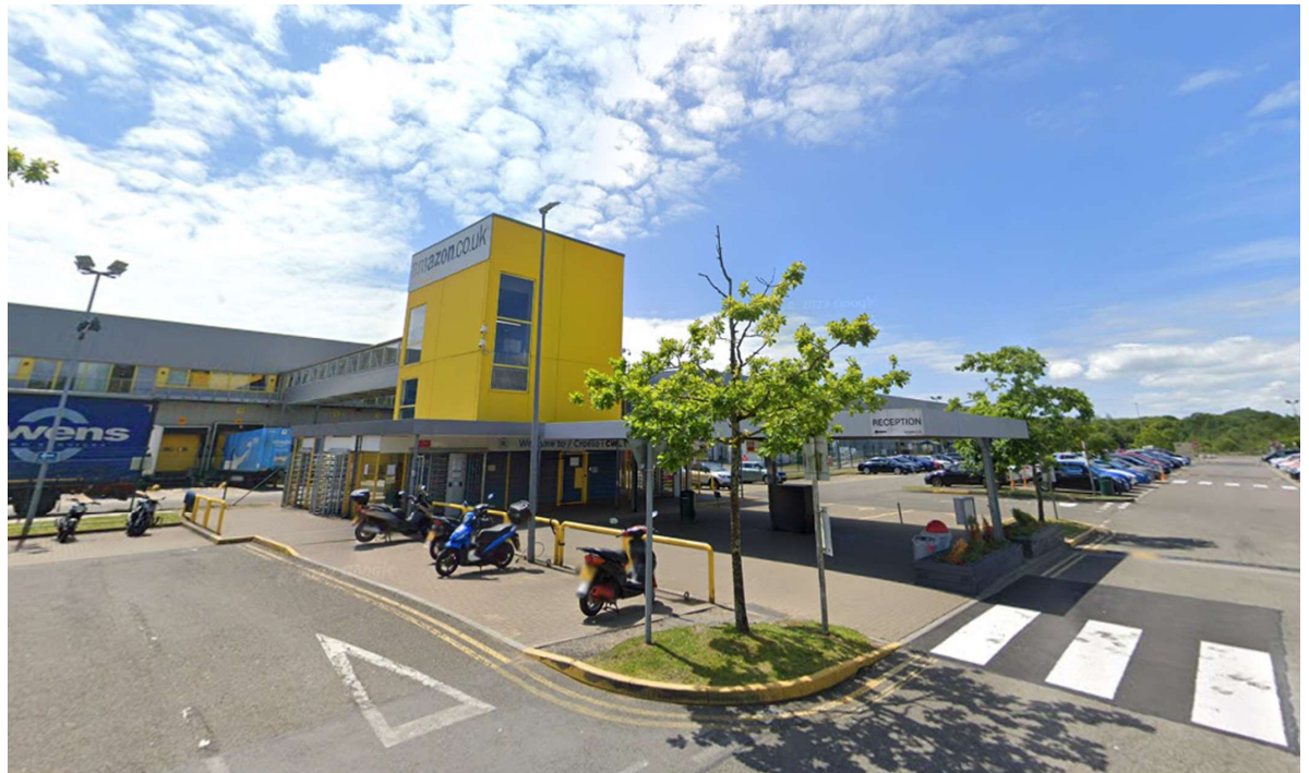
View of the existing entrance area
