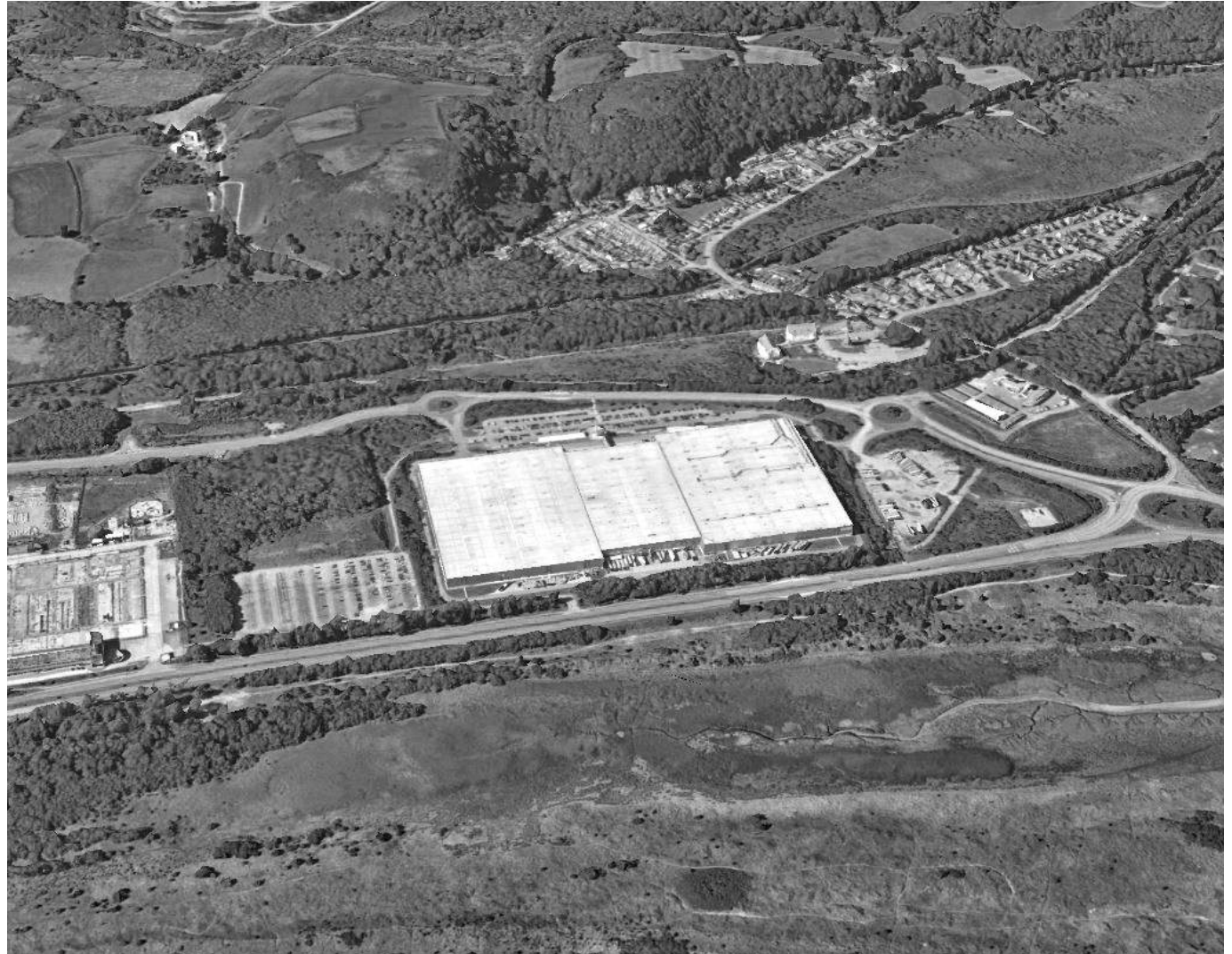
Aerial view of the Amazon CWL1 site
