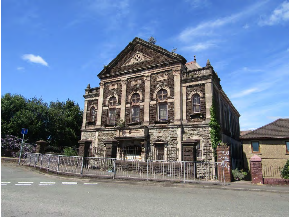
Image EDP A1.14: View north of Grade II listed Duffryn Chapel, showing its evidential and aesthetic value derived from its built fabrics and form.
