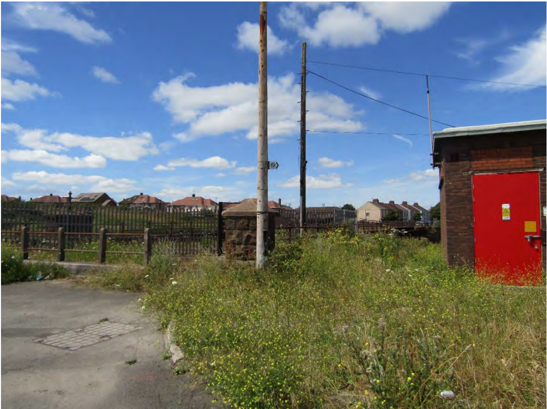
Image EDP A1.26: View west of Grade II listed Plate Girder Bridge illustrating its evidential and aesthetic values derived from its built fabrics and form.
