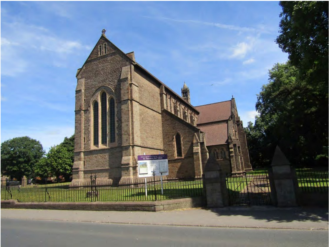
Image EDP A1.3: View north-east of the Grade II* listed Church of St Theodore, showing its evidential and aesthetic values derived from its built fabrics and form.
