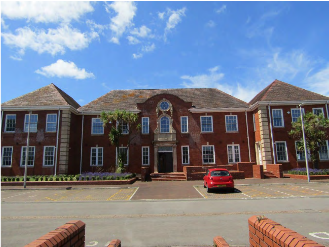
Image EDP A1.21: View west of Grade II listed Magistrates Court illustrating its evidential and aesthetic values derived from its built fabrics and form.
