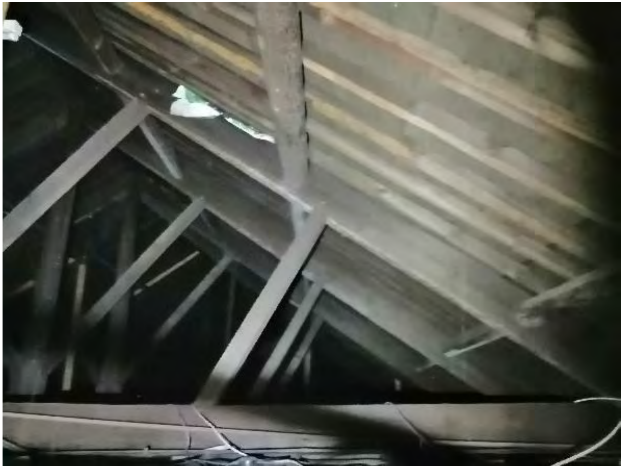
Photo 89 – Timber Roof Frameworks (Main Roof Void)
