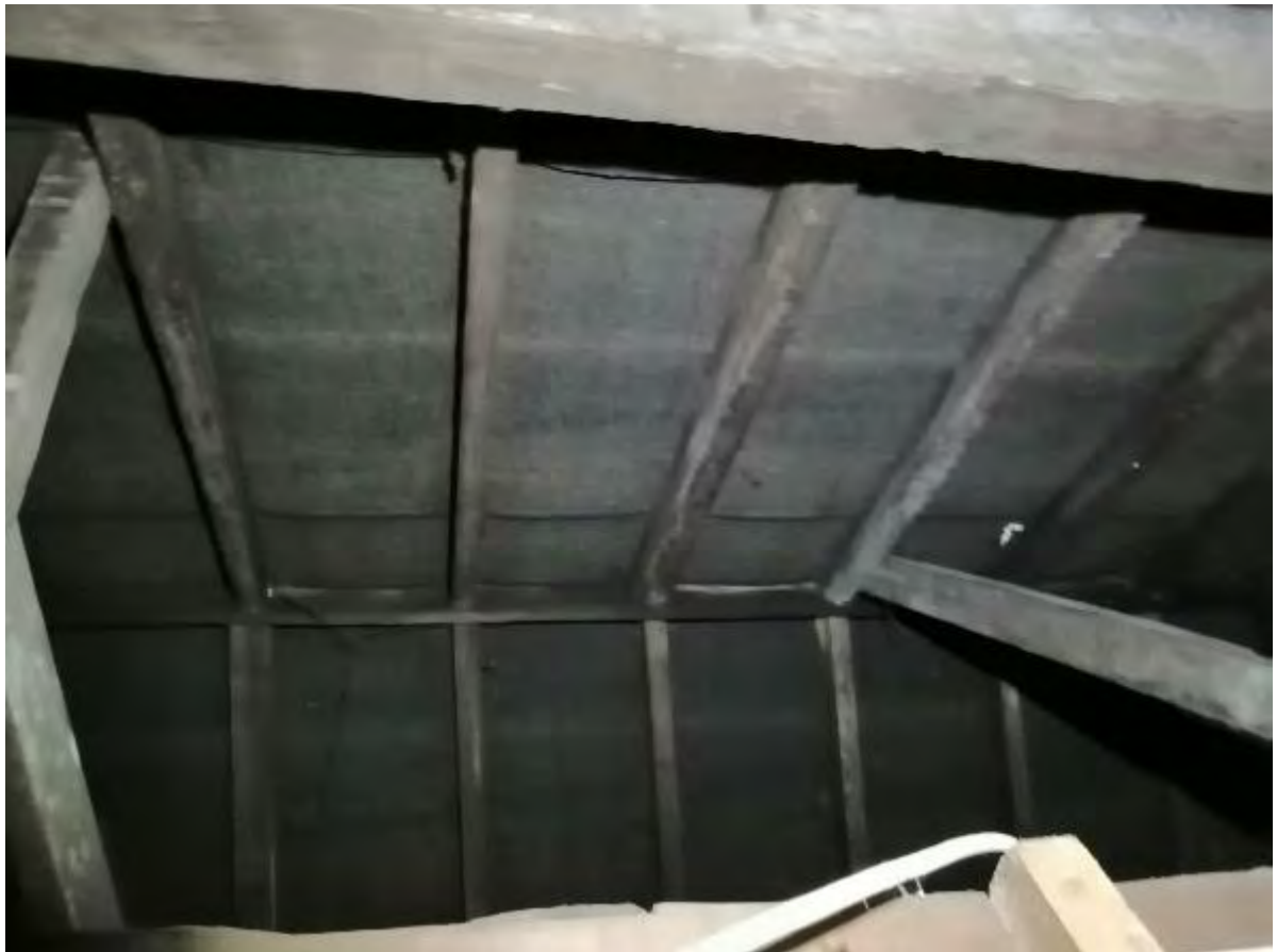
Photo 94 – Timber Roof Frameworks (Front Roof Void)
