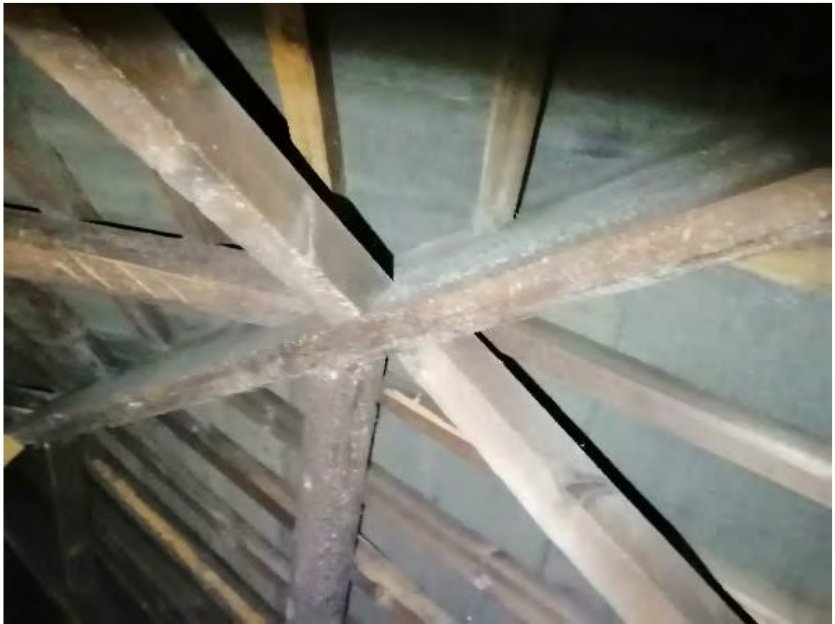
Photo 91 – Timber Roof Frameworks (Main Roof Void)
