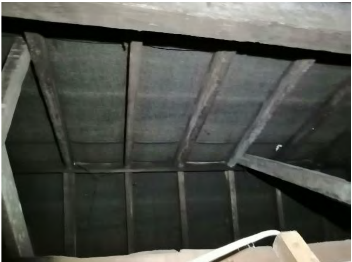
Photo 92 – Timber Roof Frameworks (Front Roof Void)
