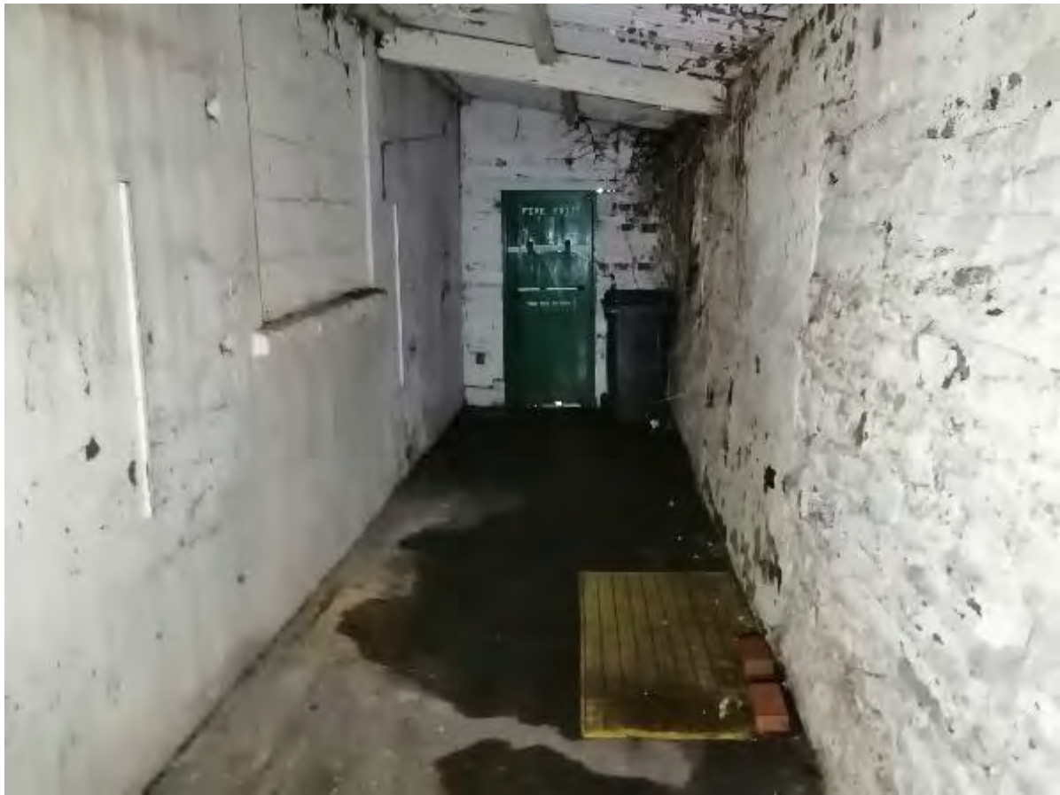
Photo 184 – Fire Exit Room
