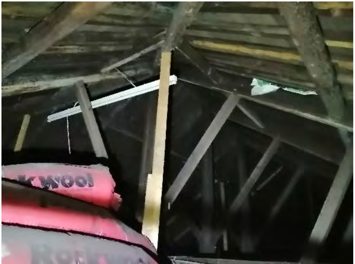
Photo 90 – Timber Roof Frameworks (Main Roof Void)
