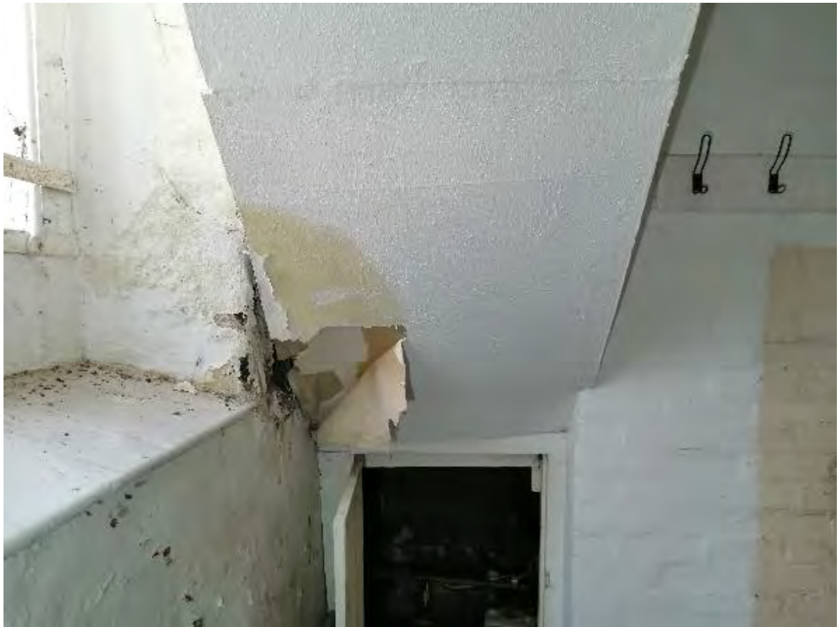
Photo 199 – Slope to Staircase (Side Room 1)
