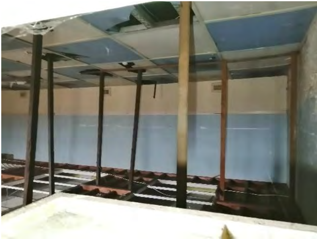
Photo 100 – Void Above Hall
