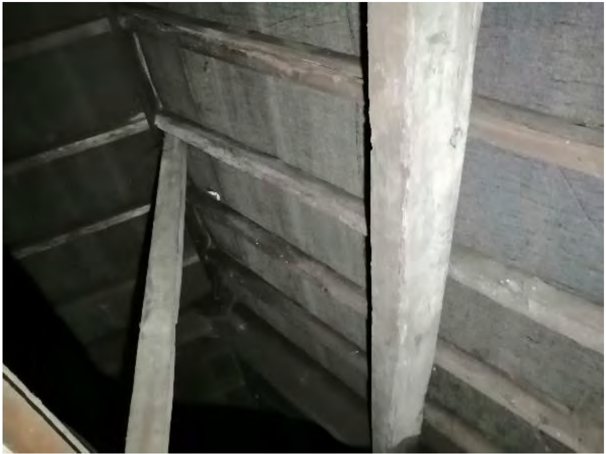
Photo 93 – Timber Roof Frameworks (Front Roof Void)
