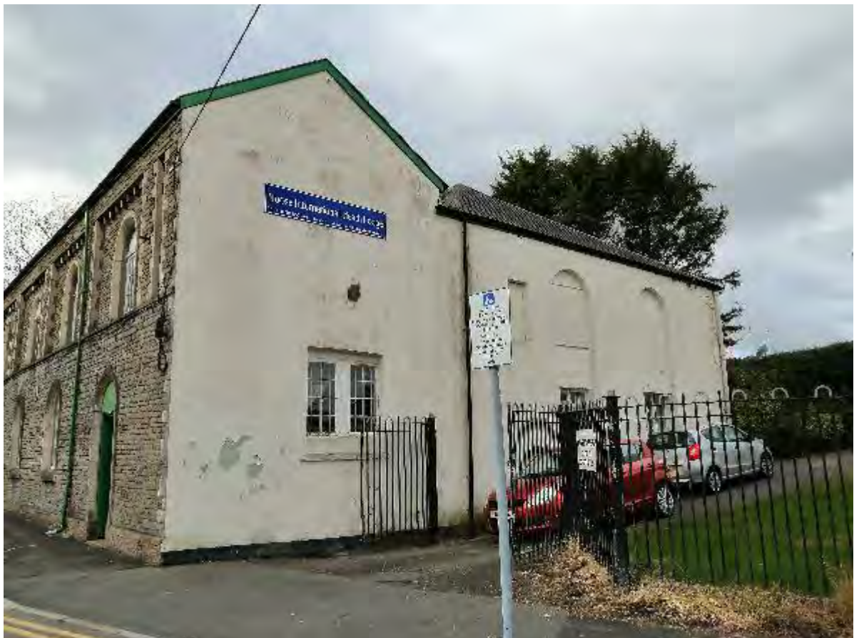
Photo 23 – Right Side Wall Elevation
