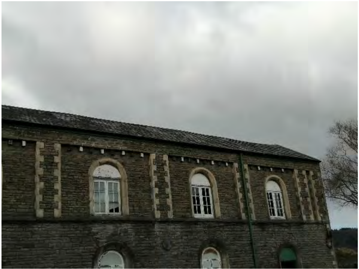
Photo 2 – Front Roof Profile (Right)
