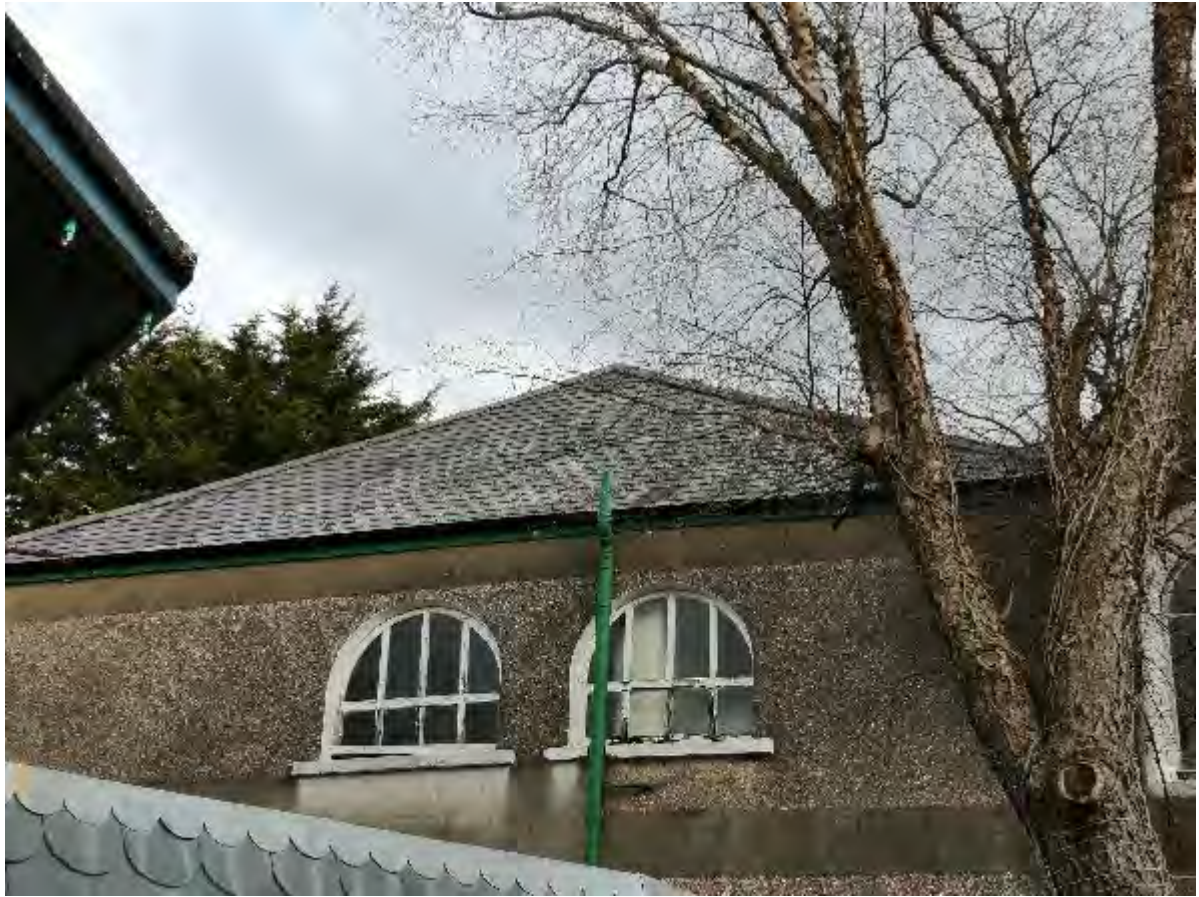
Photo 6 – Left Side Roof Profile
