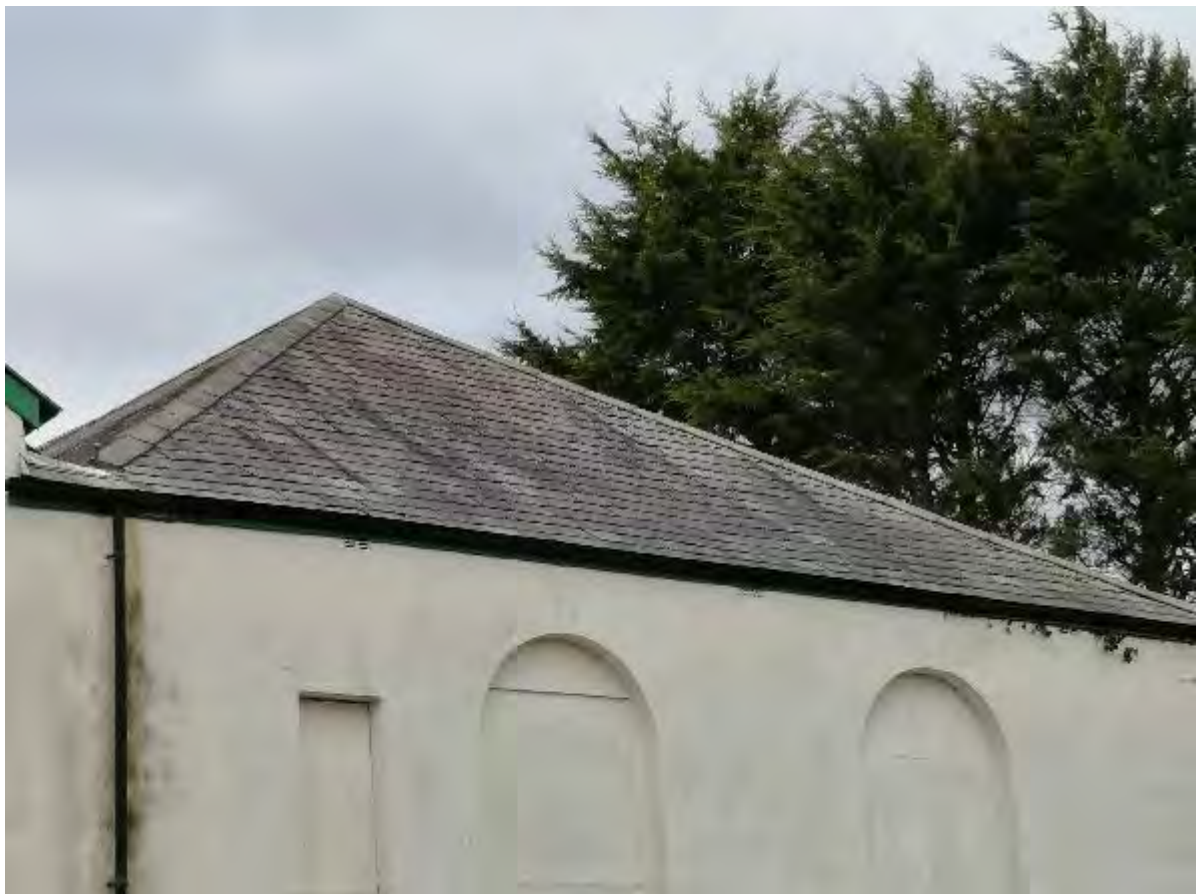
Photo 5 – Right Side Roof Profile
