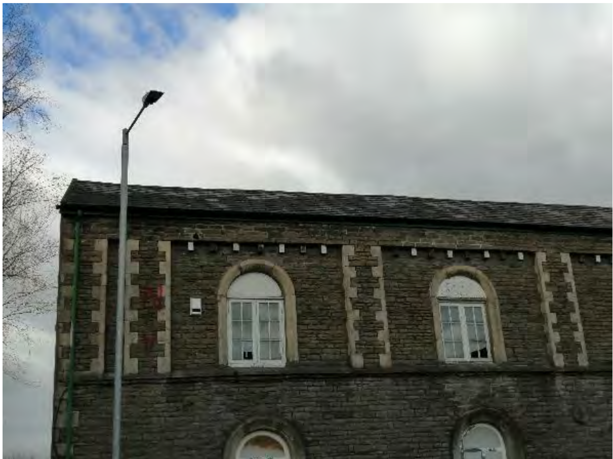
Photo 1 – Front Roof Profile (Left)
