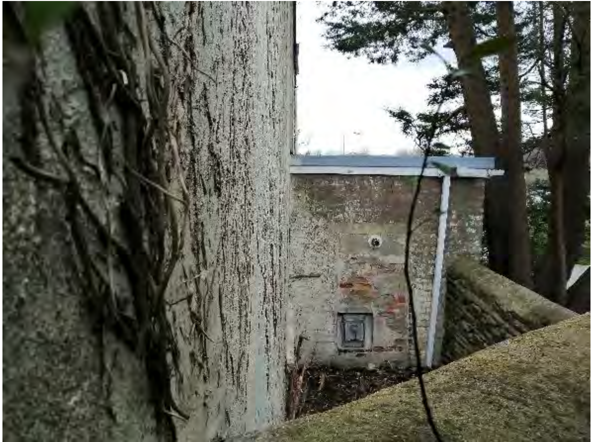
Photo 24 – Rear and Right Side Wall Elevation
