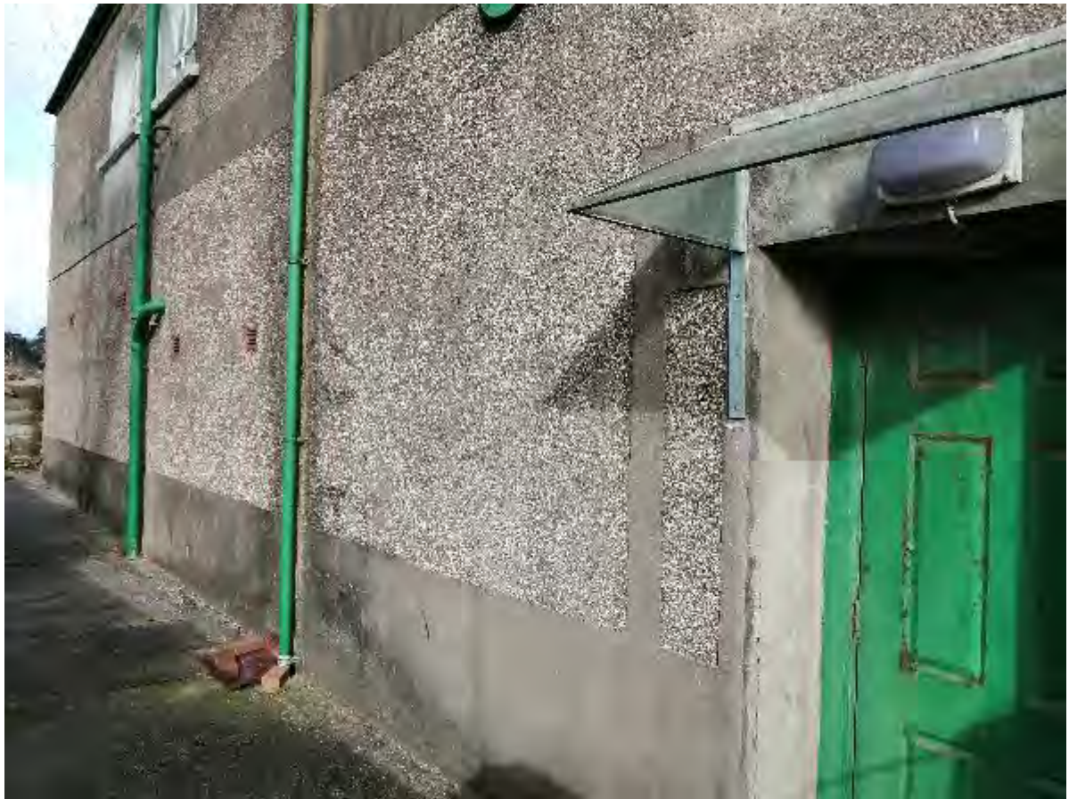
Photo 26 – Left Side Wall Elevation (Lower)
