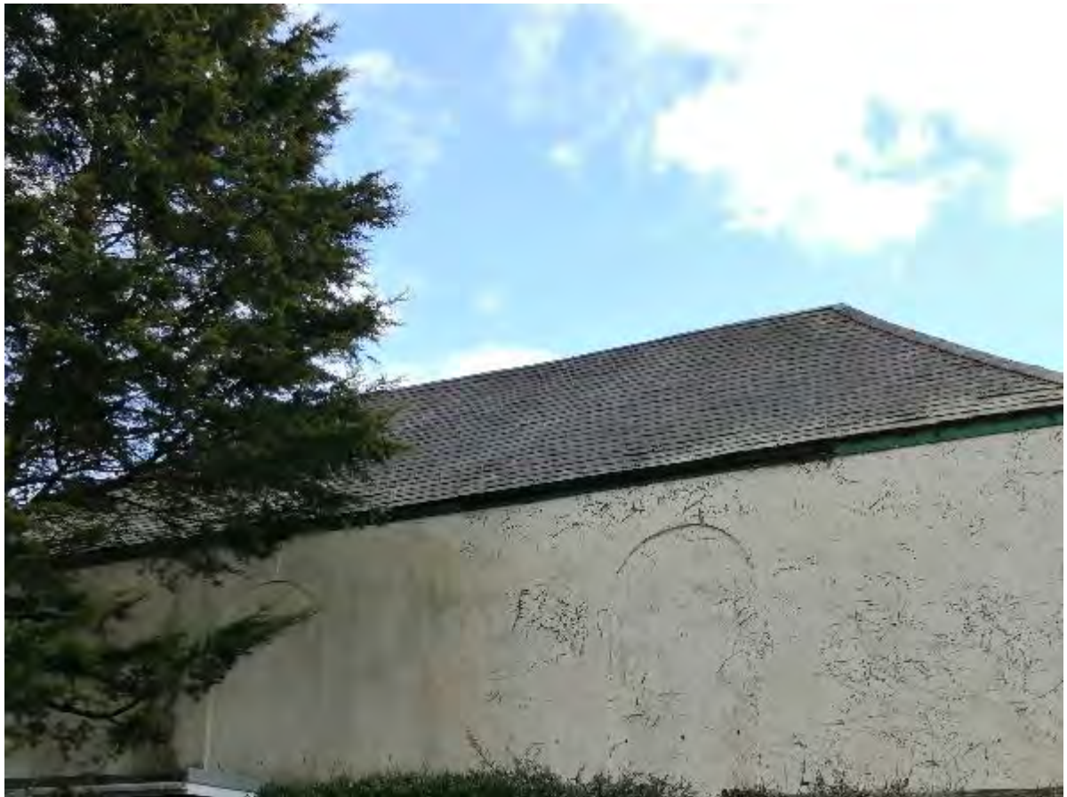
Photo 8 – Rear Roof Profile
