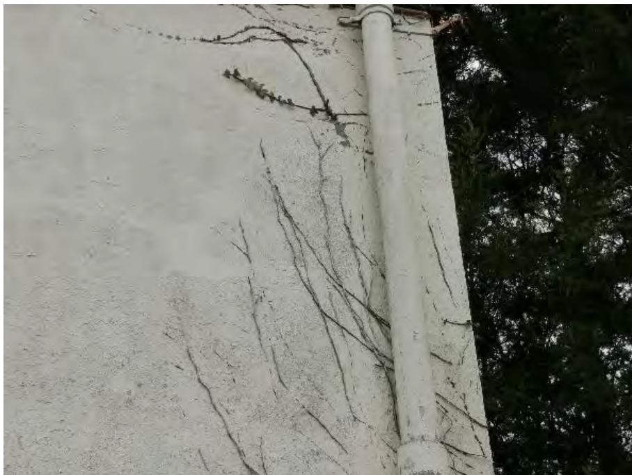
Photo 88 – Vegetation Growth (Right Wall Elevation)
