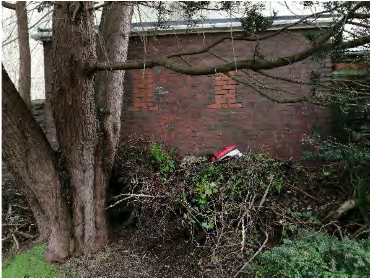
Photo 28 – Rear Wall Elevation (Lower)
