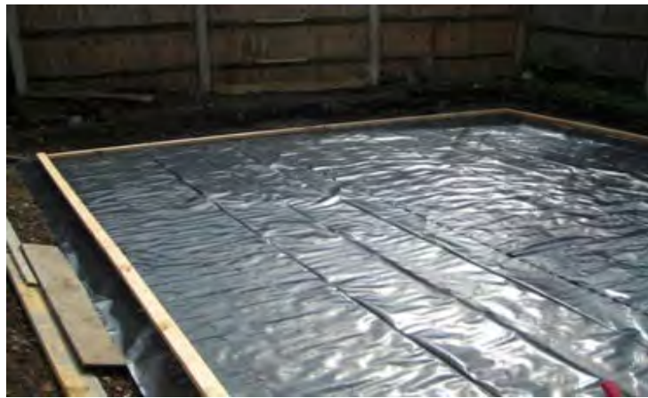
Example of a Damp Proof Membrane being installed before placement of concrete slab
