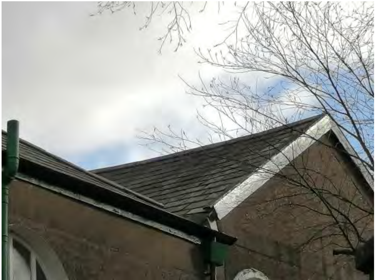
Photo 7 – Rear Roof Profile
