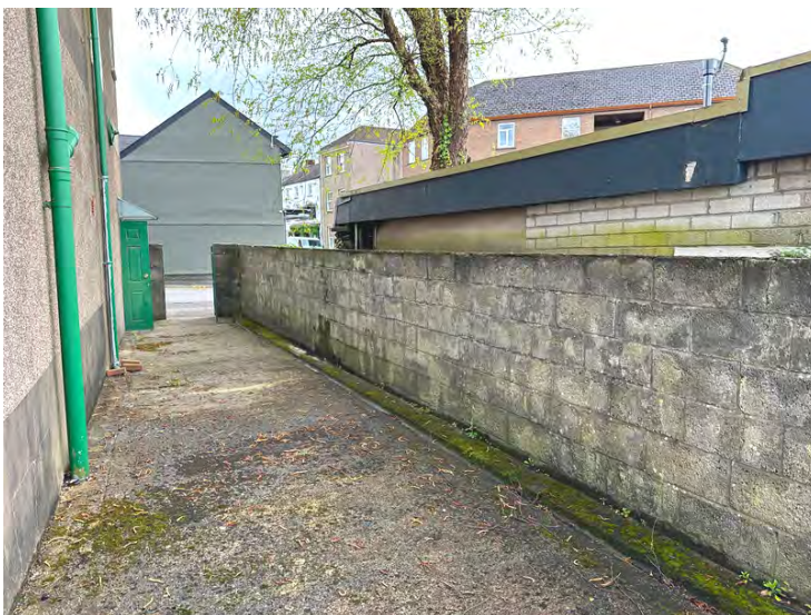
Fig 11: Access yard to west of building laid to concrete with drainage channel to perimeter.
