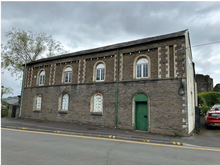
Fig 3: South elevation abuts Castle Street public highway and incorporates principal entrance
