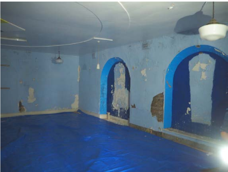
Fig 28: First floor ceremony room (within former chapel). Chapel window openings blocked and external walls covered with cementitious plaster. Boarded timber floor below tarpaulin.
