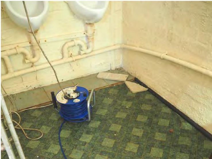
Fig 30: Male WC with modern sanitaryware, exposed pipework and contemporary finishes.
