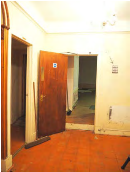
Fig 37: Entrance lobby with access to main function space beyond.
