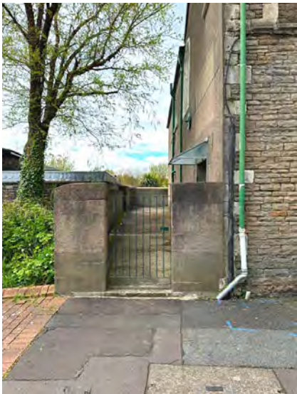
Fig 4: Secondary entrance (behind wall) to south-west corner of building, just off Castle Street
