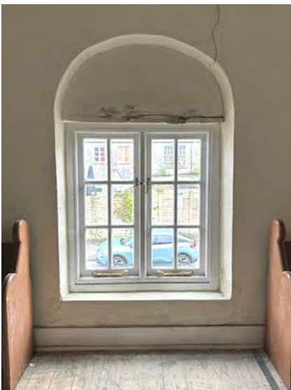
Fig 42: Modern timber casement window to south elevation, overlooking Castle Street.
