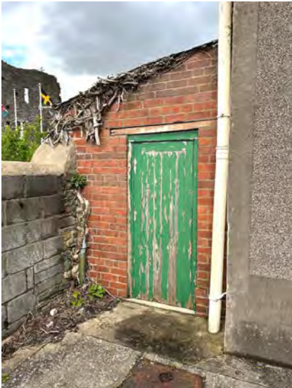
Fig 10: Lean to structure to north of former chapel with corrugated roof. Lean-to uses blockwork faced boundary wall within structure.
