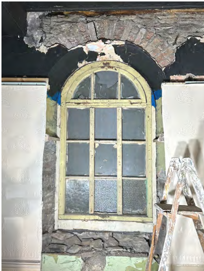
Fig 36: Removal of plasterboard in social room reveals contemporary single glazed timber window
