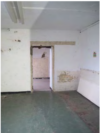
Fig 22: Secondary kitchen space leading through to kitchen store beyond.
