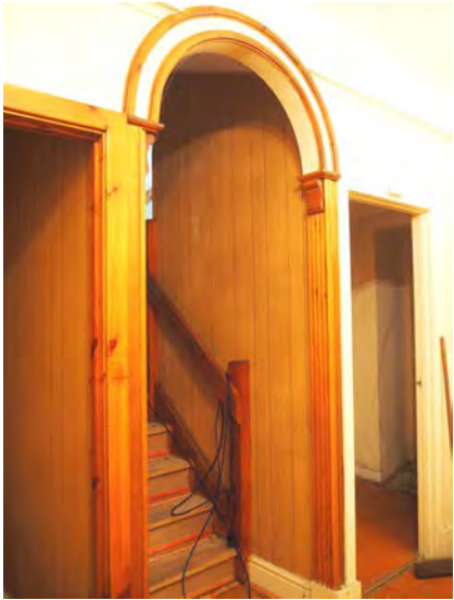
Fig 39: Timber panelling to bottom of stairs and foyer (left of frame). Female WC access (right of frame).
