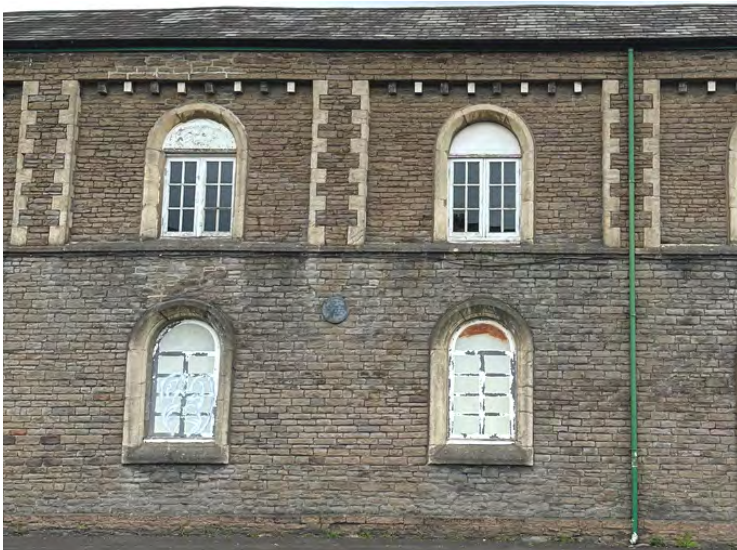
Fig 13: Each of the four bays to the south elevation incorporates a single window at both ground and first floor. At ground floor level, the existing window openings have been concealed with steel covers with painted window fenestration applied. At first floor, single glazed timber casement windows remain.
