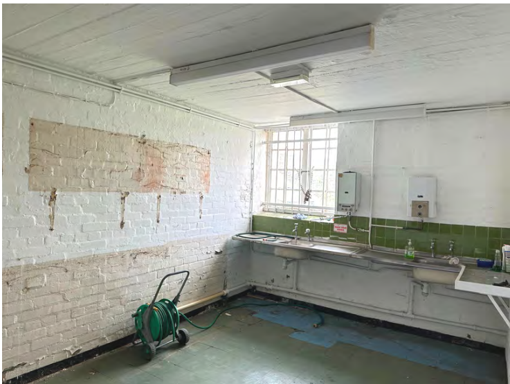
Fig 21: Kitchen adjacent to function space. Equipment removed with shuttered concrete ceiling, painted brick walls and vinyl tile floor evident. Metal windows to east elevation.
