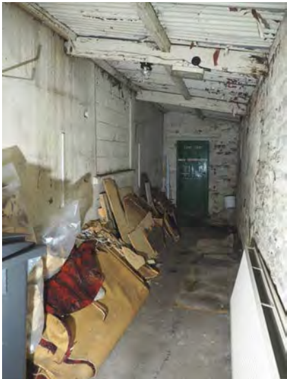
Fig 26: External store (west) with fire escape & blocked up window chapel window opening.
