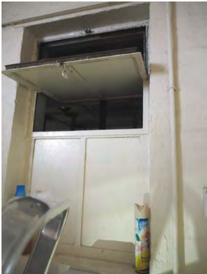
Fig 31: Internal metal window between Male WC and roof void (over ground floor function room).
