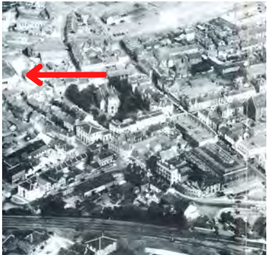
Fig 48: 1950's aerial image of Neath illustrating the building as a fire station (refer to large door opening in west elevation)
