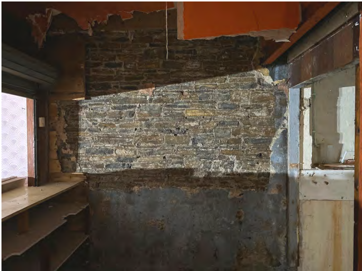
Fig 25: Modern cementitious plaster surface behind bar area removed to expose solid stone external wall below.
