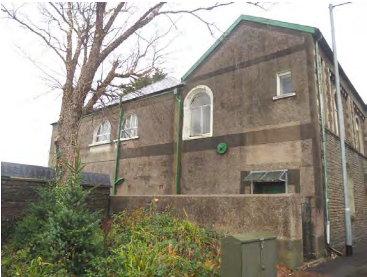
Fig 7: Former Wesleyan chapel structure with hipped slate roof to the northern part of the site (LHS of photograph) and later, gabled structure to the south and fronting onto Castle Street (RHS of photograph).
