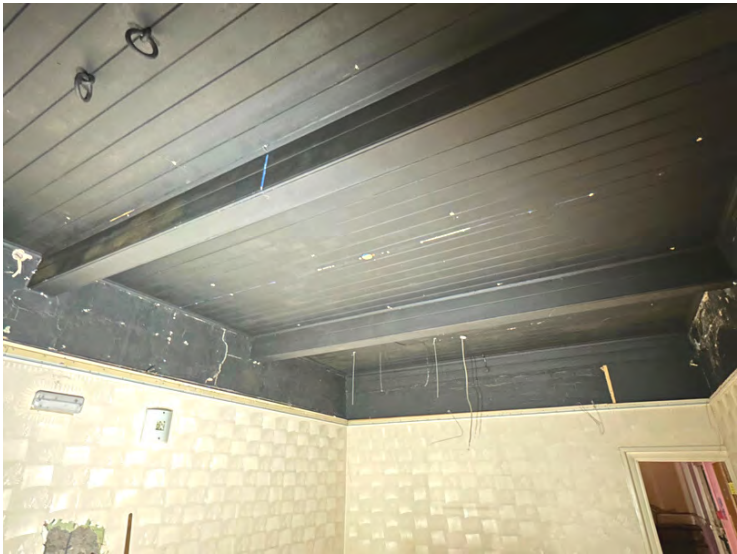
Fig 35: Social Room ceiling following removal of lay-in-grid - painted timber boarding revealed.
