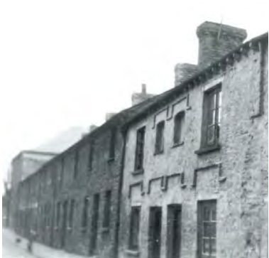
Fig 47: 1930's image of 'The Latt' with the Friends Meeting House in the background
