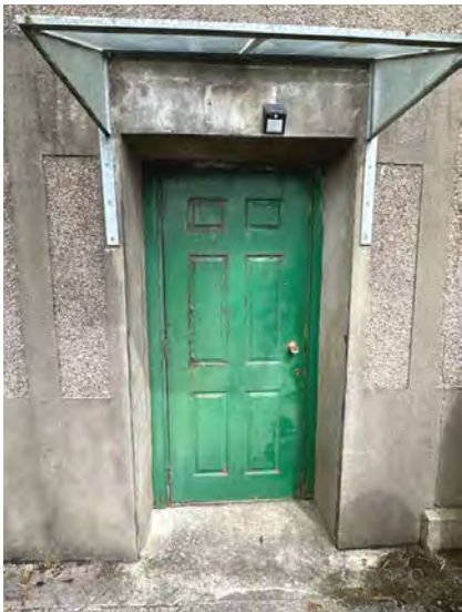
Fig 16: Secondary entrance located in yard to west elevation. contemporary steel door with modern galvanised steel framed canopy over.
