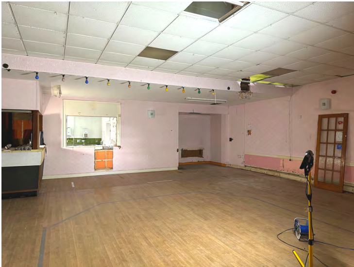
Fig 12: Main function space with access/view through serving hatch to kitchen. Surfaces include lay-in-grid ceiling, cementitious plaster walls/wallpaper finish and sprung timber floor.
