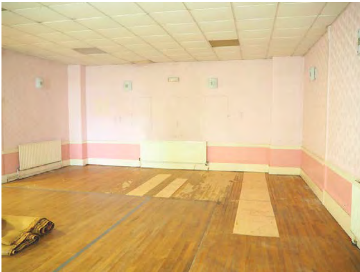
Fig 14: Former fire station entrance to east wall, Floor includes gentle slope towards former door. Modern panelled radiators fitted.
