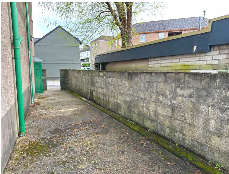
Fig 6: Access yard to west of building laid to concrete with drainage channel to perimeter.
