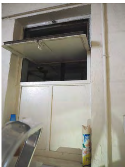
Fig 26: Internal metal window between Male WC and roof void (over ground floor function room).
