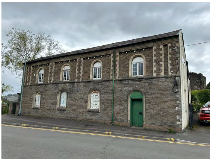
Fig 4: South elevation abuts Castle Street public highway and incorporates principal entrance
