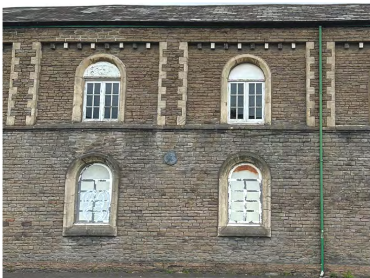
Fig 10: Each of the four bays to the south elevation incorporates a single window at both ground and first floor. At ground floor level, the existing window openings have been concealed with steel covers with painted window fenestration applied. At first floor, single glazed timber casement windows remain.
