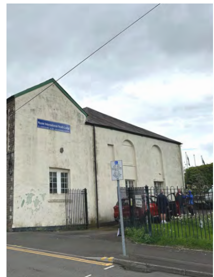
Fig 7: Driveway and gardens to the east of the building are under separate ownership.
