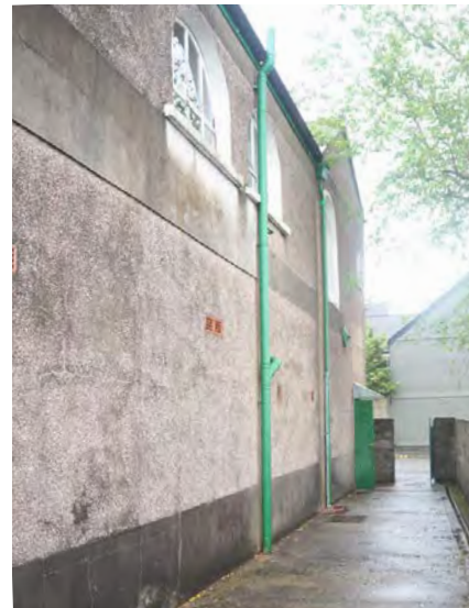
Fig 9: Canterbury Spar (Durite) finish to west elevation.
