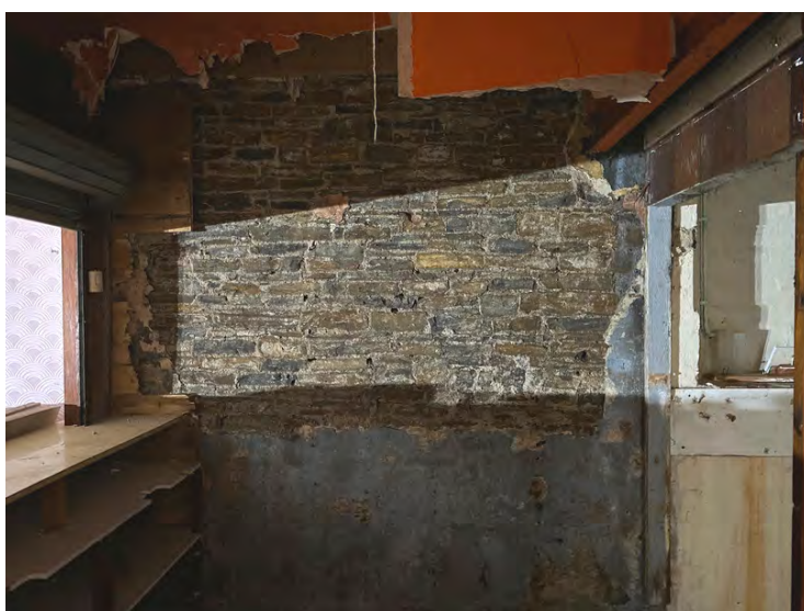
Fig 20: Modern cementitious plaster surface behind bar area removed to expose solid stone external wall below.
