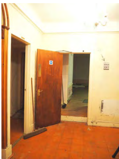
Fig 32: Entrance lobby with access to main function space beyond.
