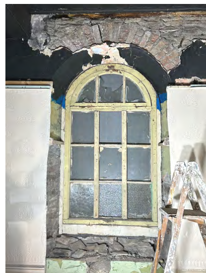
Fig 31: Removal of plasterboard in social room reveals contemporary single glazed timber window
