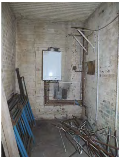
Fig 22: External store (east) housing gas fired boiler.
