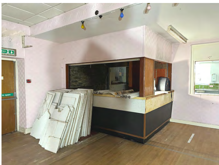
Fig 18: stained timber and melamine bar enclosure to north east corner of function room, leading to bar store and kitchen beyond.
