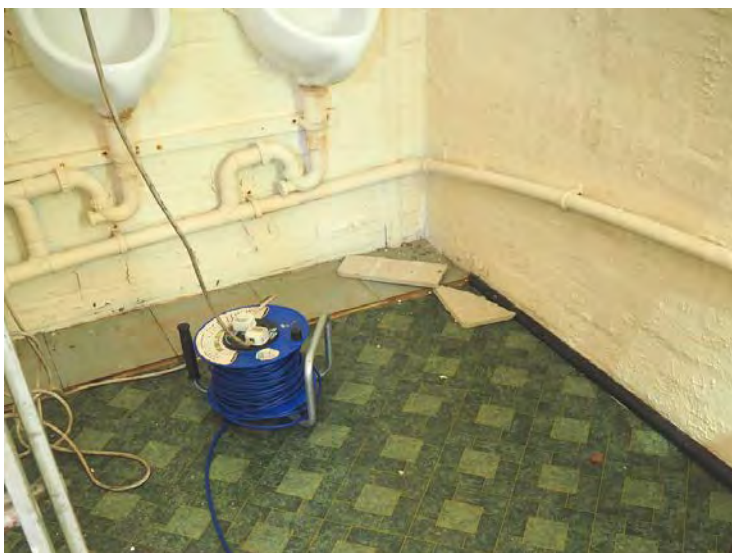
Fig 25: Male WC with modern sanitaryware, exposed pipework and contemporary finishes.
