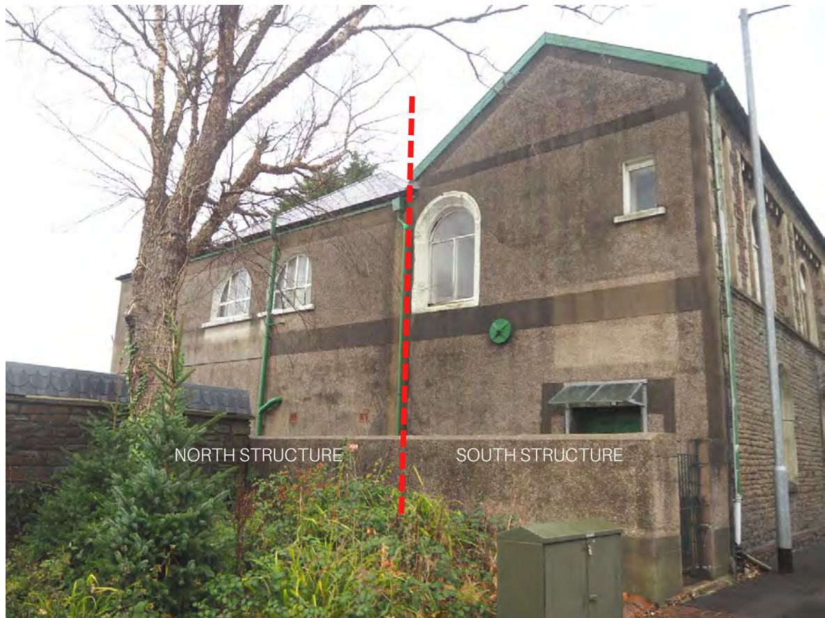
Fig 1: Former Wesleyan chapel structure with hipped slate roof to the northern part of the site (LHS of photograph) and later, gabled structure to the south and fronting onto Castle Street (RHS of photograph).
