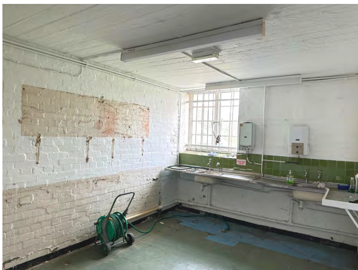
Fig 16: Kitchen adjacent to function space. Equipment removed with shuttered concrete ceiling, painted brick walls and vinyl tile floor evident. Metal windows to east elevation.
