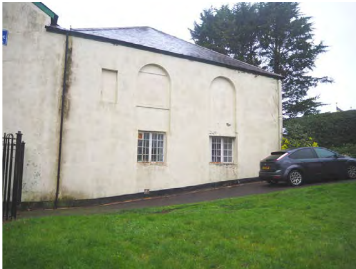
Fig 8: Sand and cement render to east elevation, paint finish.
