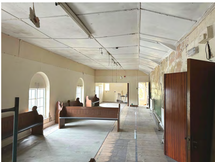
Fig 35: First floor Hall within extension structure overlooking Castle Street.
