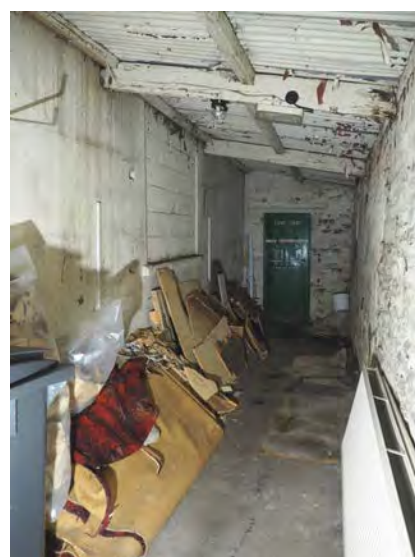
Fig 21: External store (west) with fire escape & blocked up window chapel window opening.
