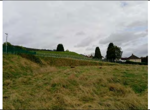
Plate 8: view from the centre of the site looking north towards northern most playing field and soil batters.
