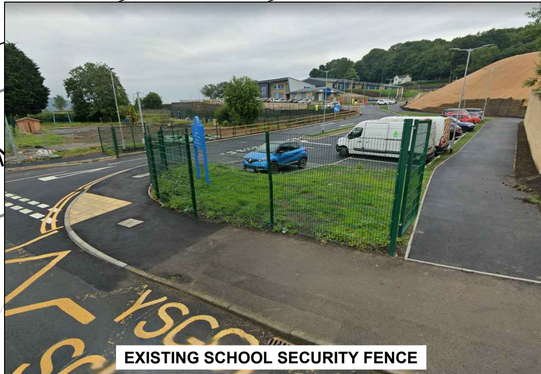
EXISTING SCHOOL SECURITY FENCE
