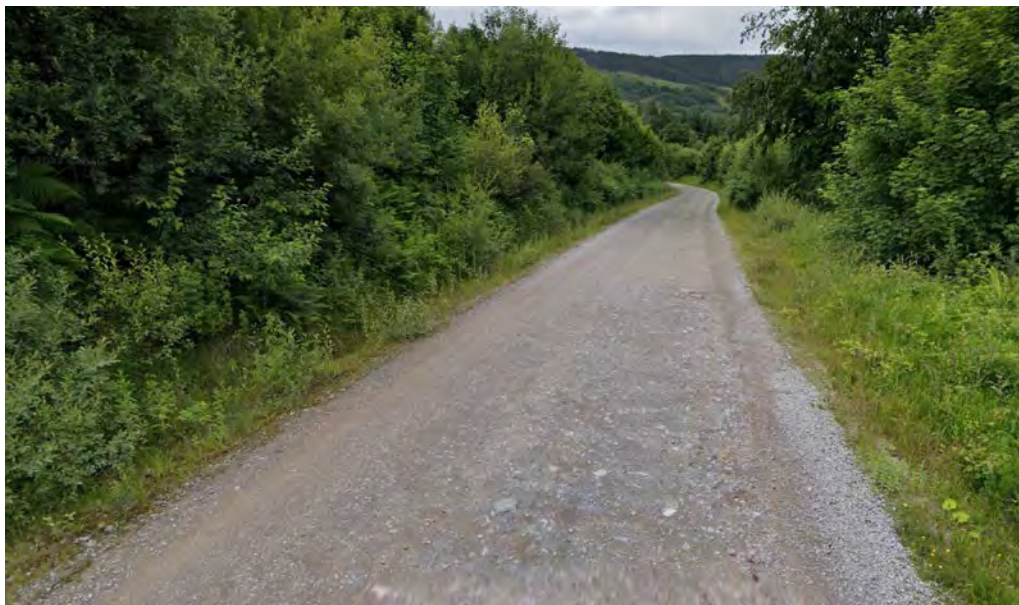
Figure 6 Stone Section of Forestry Road
