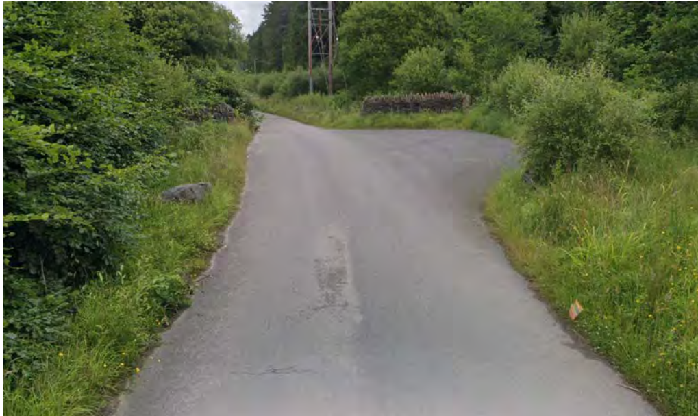
Figure 5 Asphalt Section of Forestry Road
