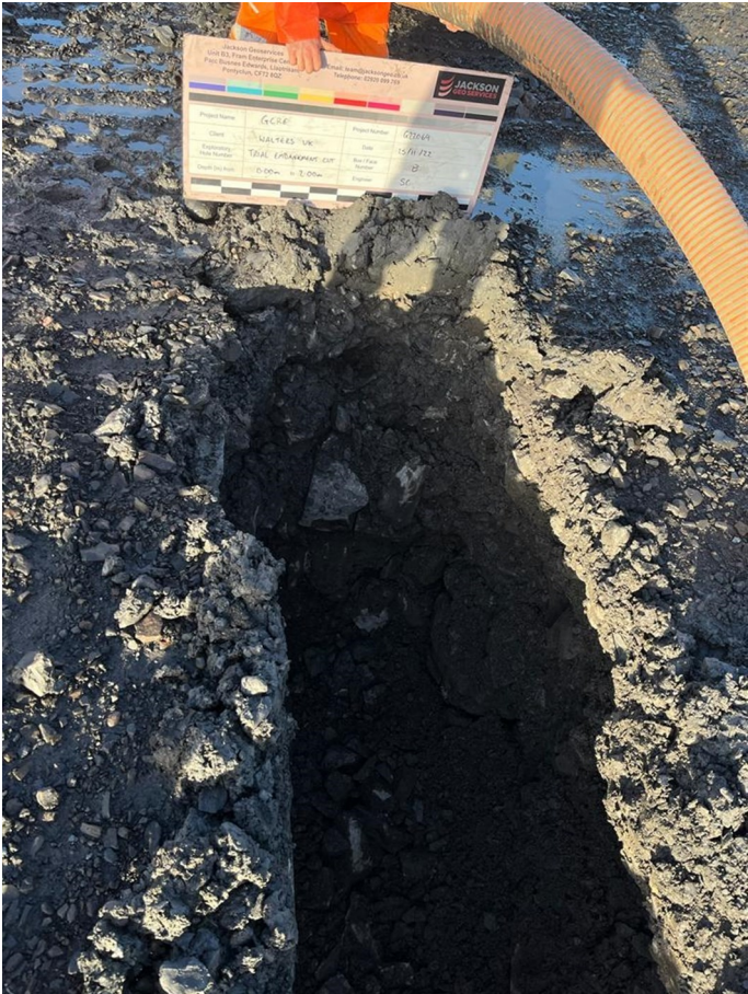
Trial Embankment Cut - Face B
