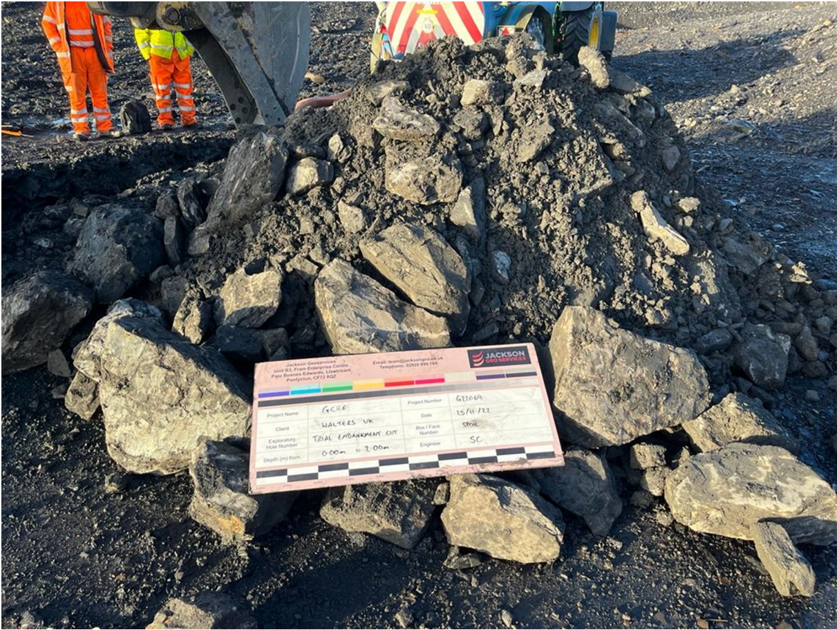
Trial Embankment Cut - Spoil
