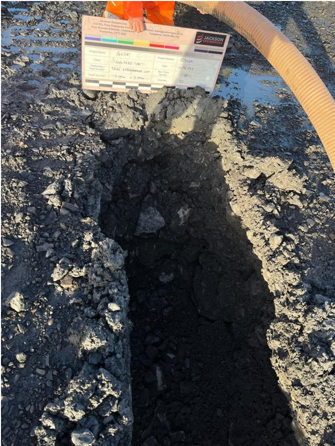
Trial Embankment Cut - Face B
