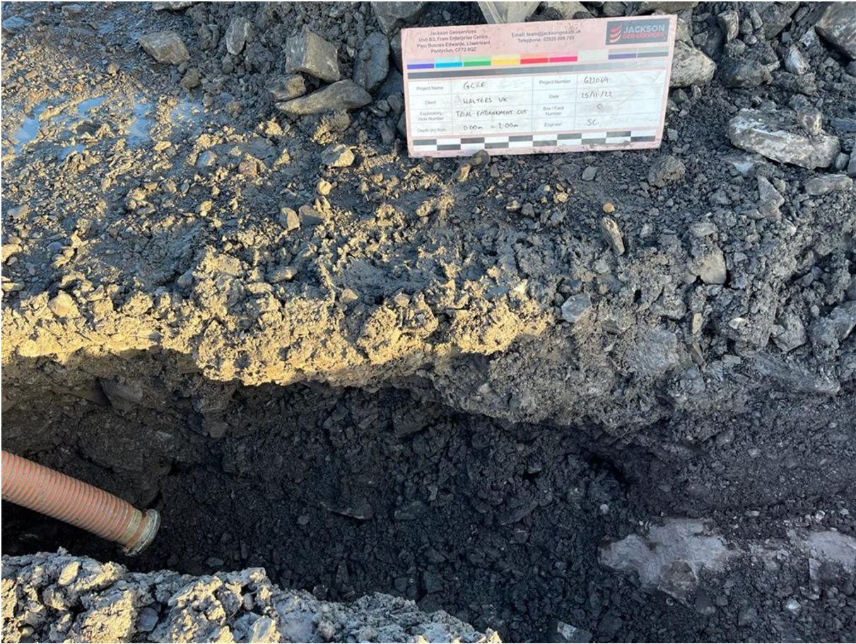
Trial Embankment Cut - Face C
