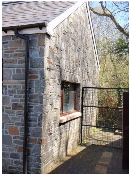
Photo 7.1 – South West Elevation
