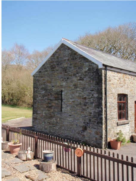
Photo 9.1 – North West Elevation
