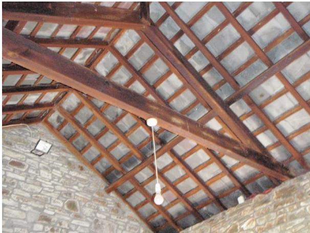
Photo 6.1 – Original Barn Roof
