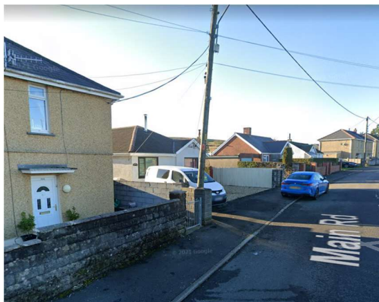
Street View of Proposed Access Point
