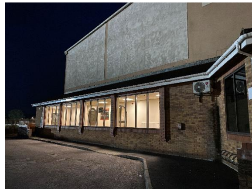
Figure 4: South side (western end)
