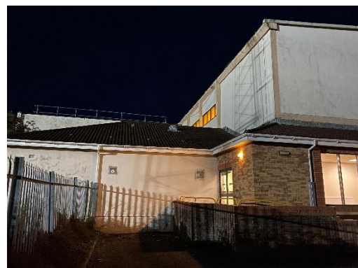
Figure 6: West side (NW corner)
