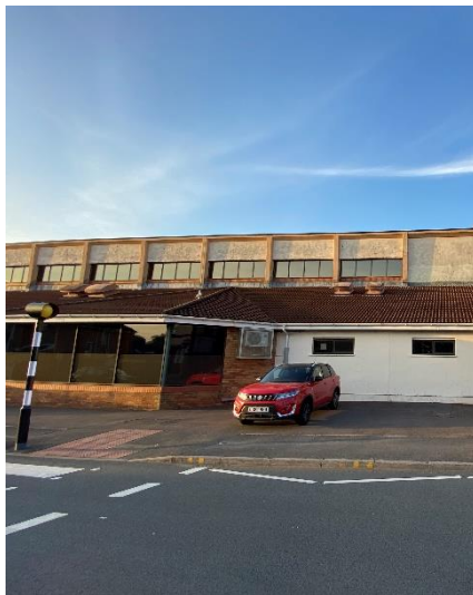
Figure 3: South side of leisure centre from Dyfed Road (SE)
