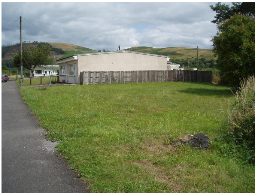
Views of the Rofton nonstandard construction bungalows
