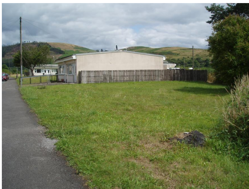
Typical views of the amenity areas and bungalows
