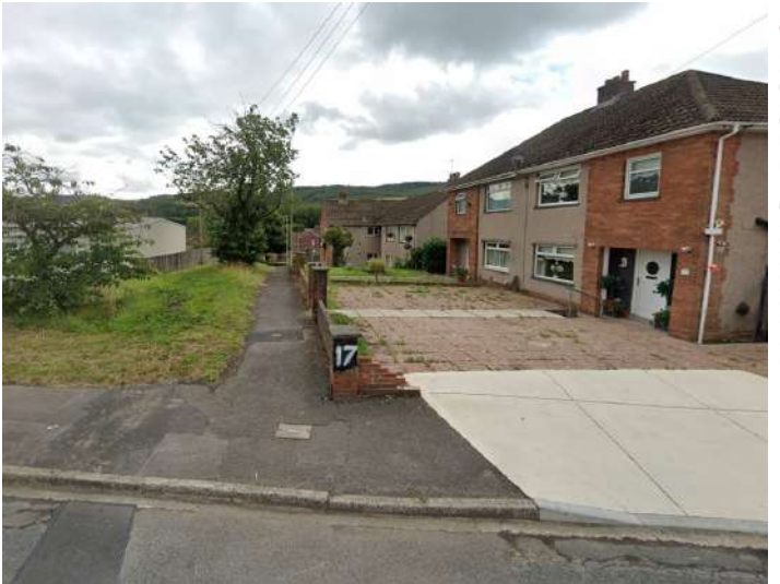
Site's nearest residential receptor, at the north-western boundary. In respect of residential amenity, a respectful separation distance is evident.
