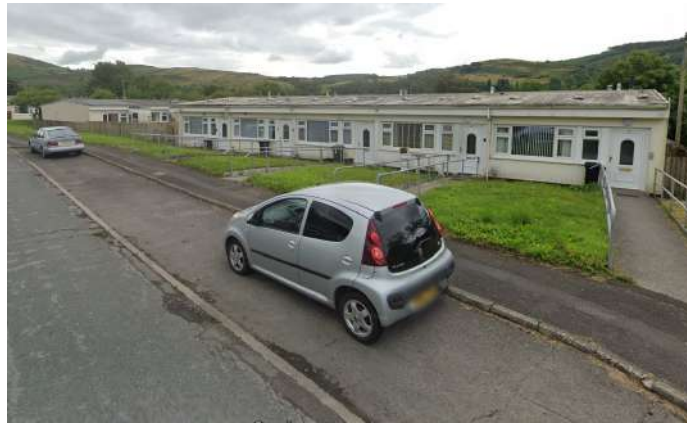
Bungalows deteriorating in appearance and lack of resident parking, which is currently provided in the form of on-street laybys.
