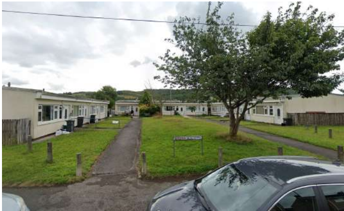
Existing context of Heol Crwys - one-storey bungalows.
