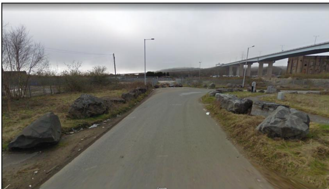
Figure 15.0 – Site Entrance (Google Image)
