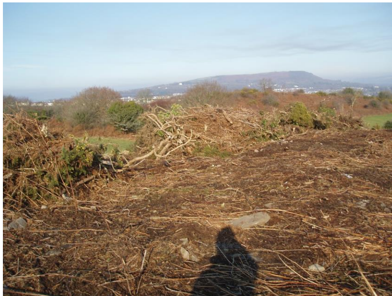
Machine cleared are east of TN6 hedge bank
