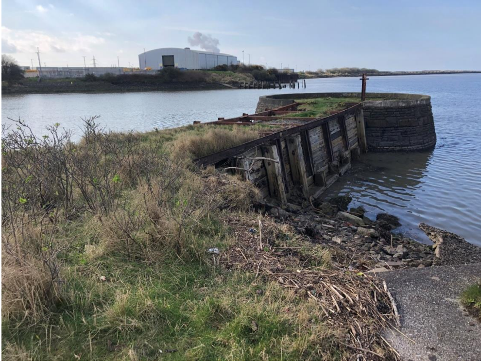
Figure 20 - the North Jetty
