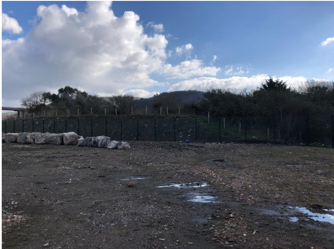
Figure 9 - recently constructed earth bund to south-east boundary
