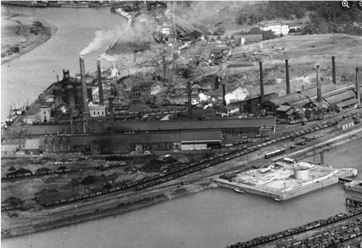
Figure 6 - aerial view of c.1950, the Coke Works demolished
