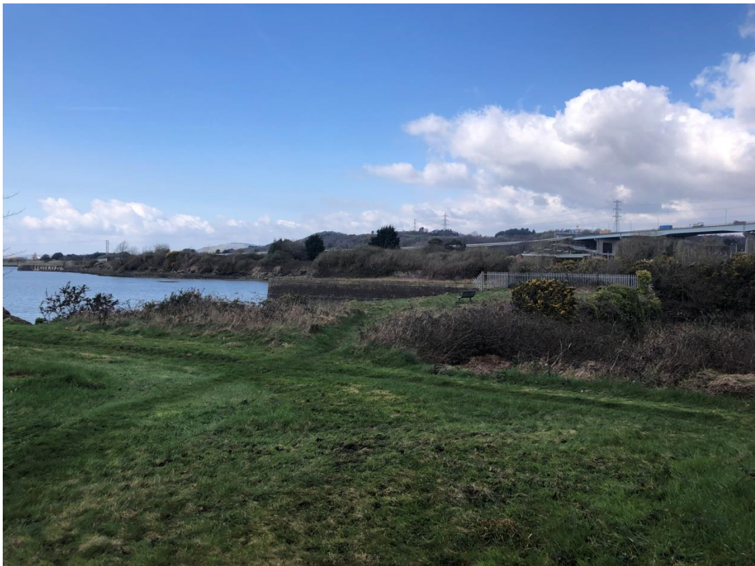
Figure 21 - site viewed from the south-east from Briton Ferry Dock with the North Jetty visible to the left
