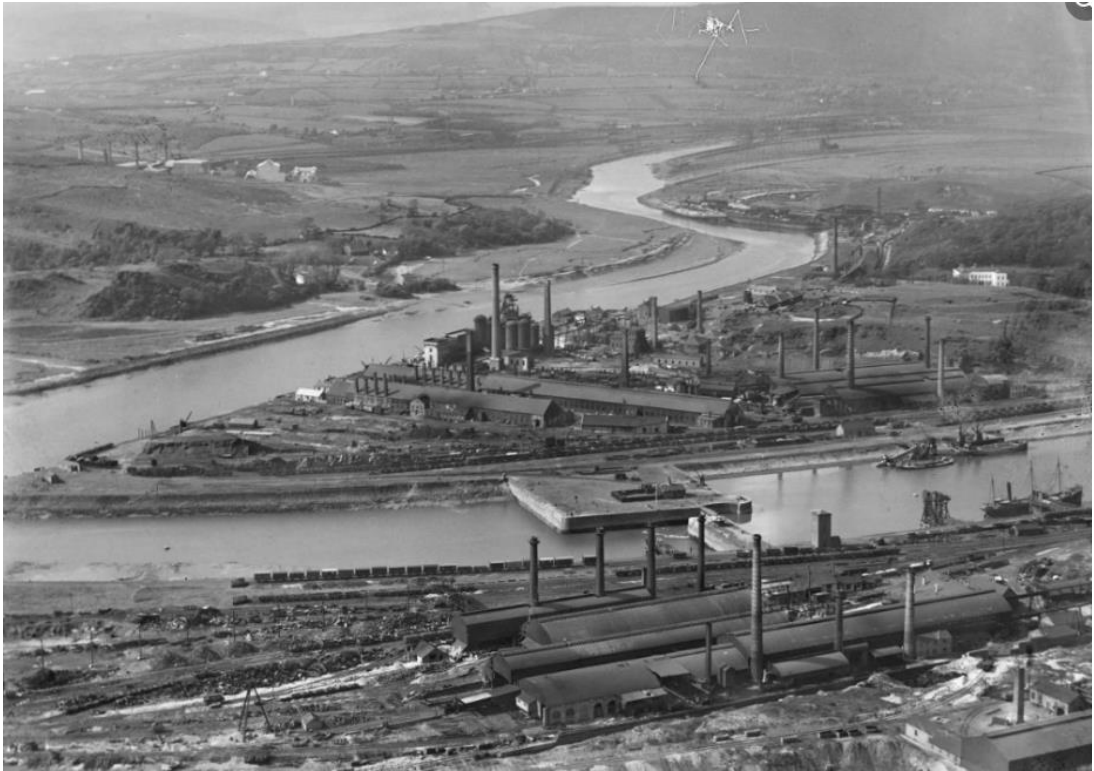
Figure 2 - aerial view of 1921 looking towards site from south-east. Briton Ferry Dock in the foreground.
