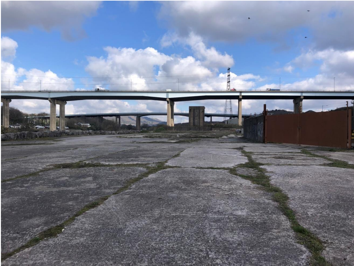
Figure 8 - site looking north towards listed Engine House and M4 Bridge
