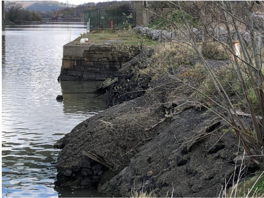
Figure 10 - Victorian revetment to north-west corner of site
