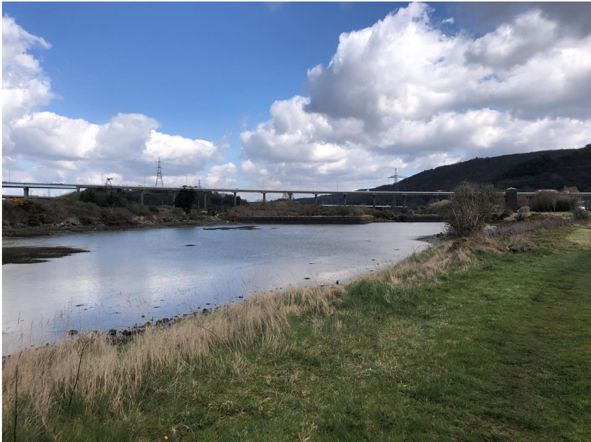
Figure 13 - Brunel's Briton Ferry Dock viewed from the south-west
