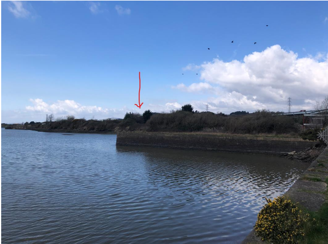
Figure 14 - view from SAM looking west towards site (marked with arrow). The listed North Jetty is visible to the left edge of the photo
