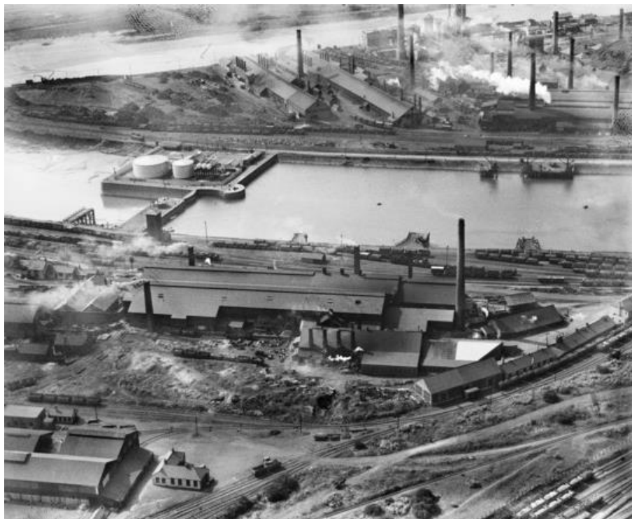
Figure 3 - aerial view from south of 1935 showing Cambrian Cokeworks, Gwalia and Victoria Tinplate Works and Briton Ferry Steelworks
