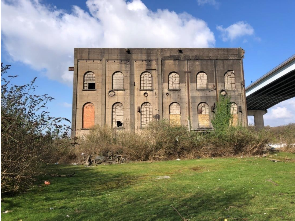
Figure 23 - Briton Ferry Ironworks Engine House
