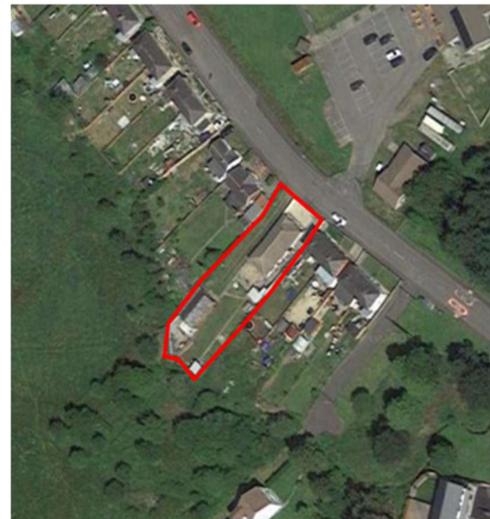
Aerial View of the site (site in red)
