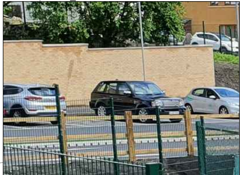
EXISTING SCHOOL RETAINING WALL
