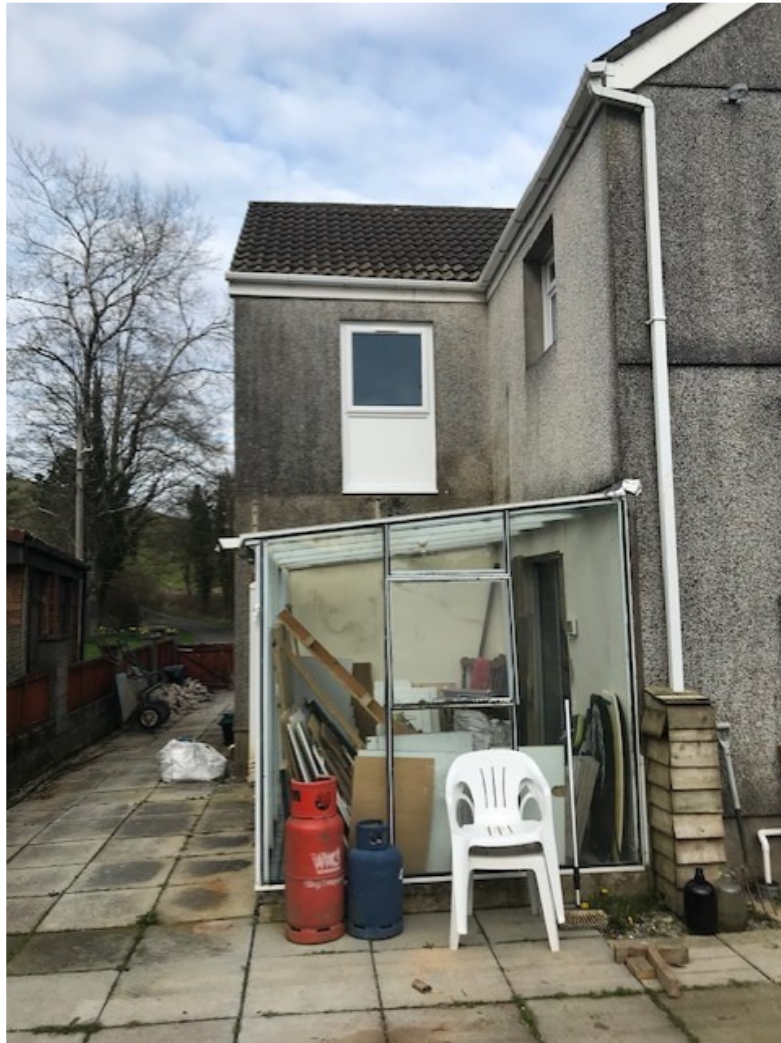
Photograph shows rear view of property with access door to first floor unit replaced with new window and external staircase removed.
