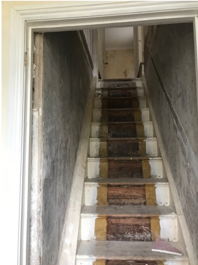
Photograph shows original internal staircase with opening reinstated.
