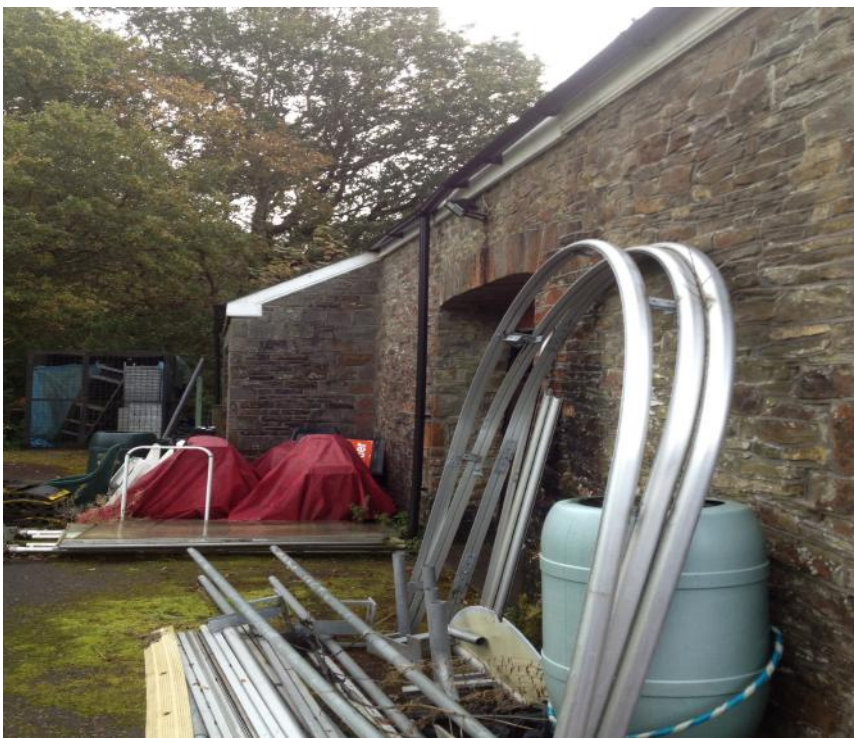
Existing north facing elevation of barn number 1.
