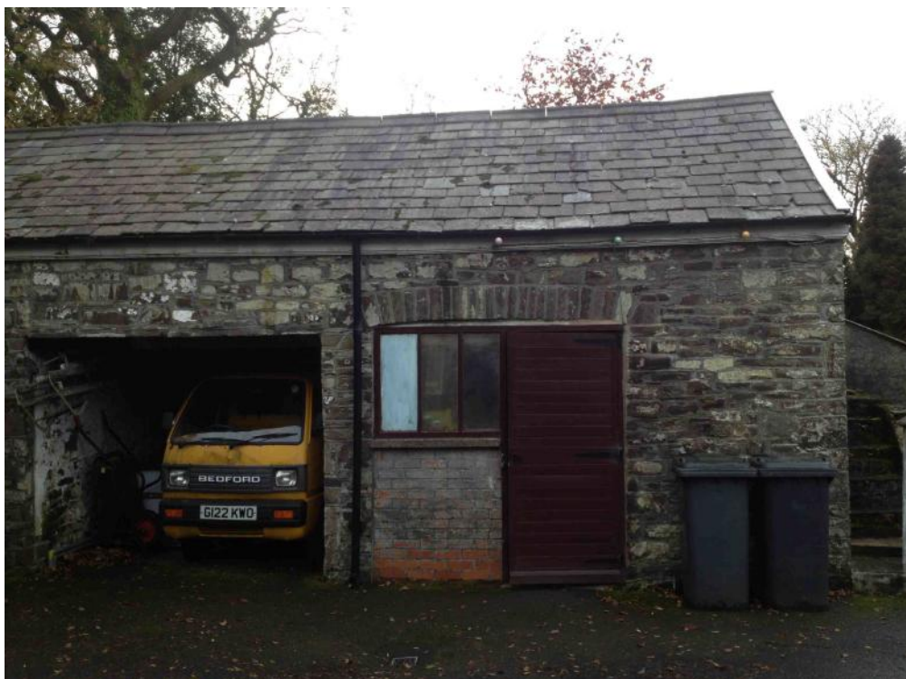
Existing north facing elevation of barn number 2.
