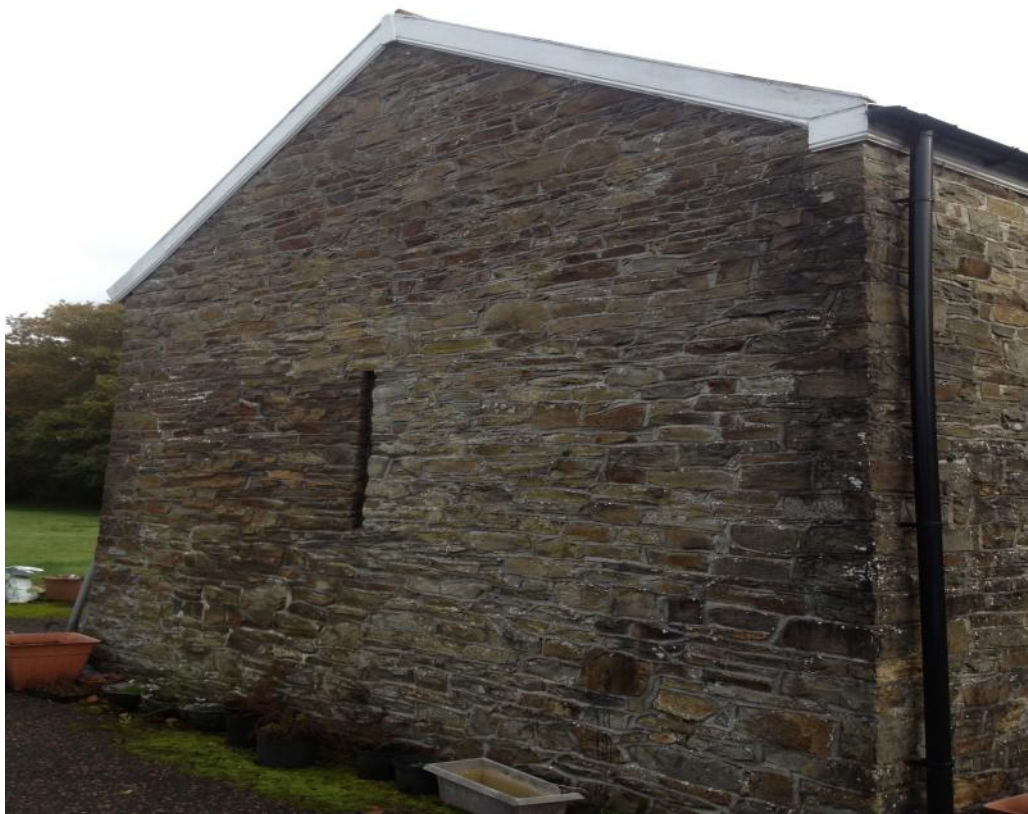
Existing west facing elevation of barn number 1.
