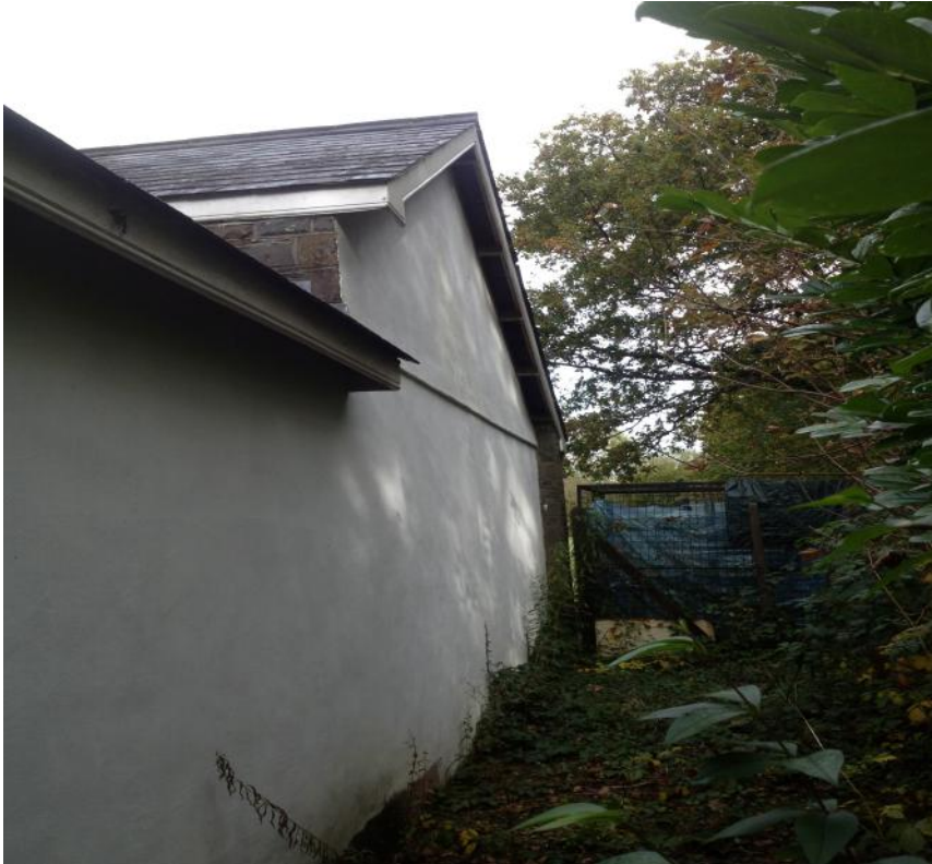
Existing east facing elevation of barn number 1.
