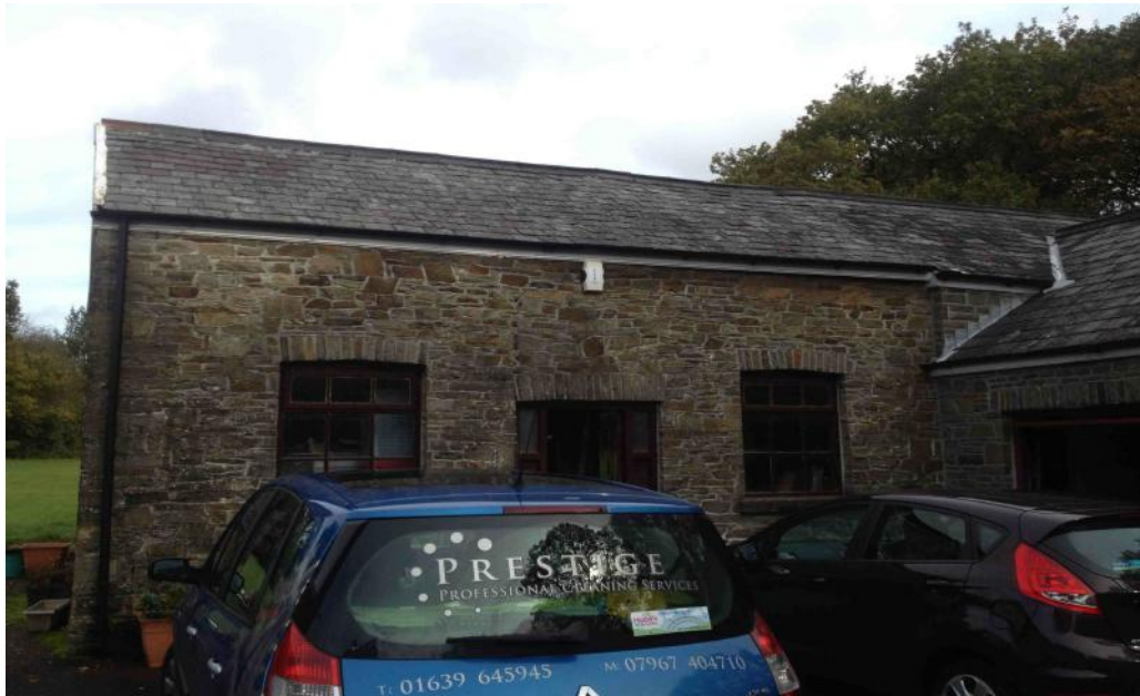
Existing south facing elevation of barn number 1.
