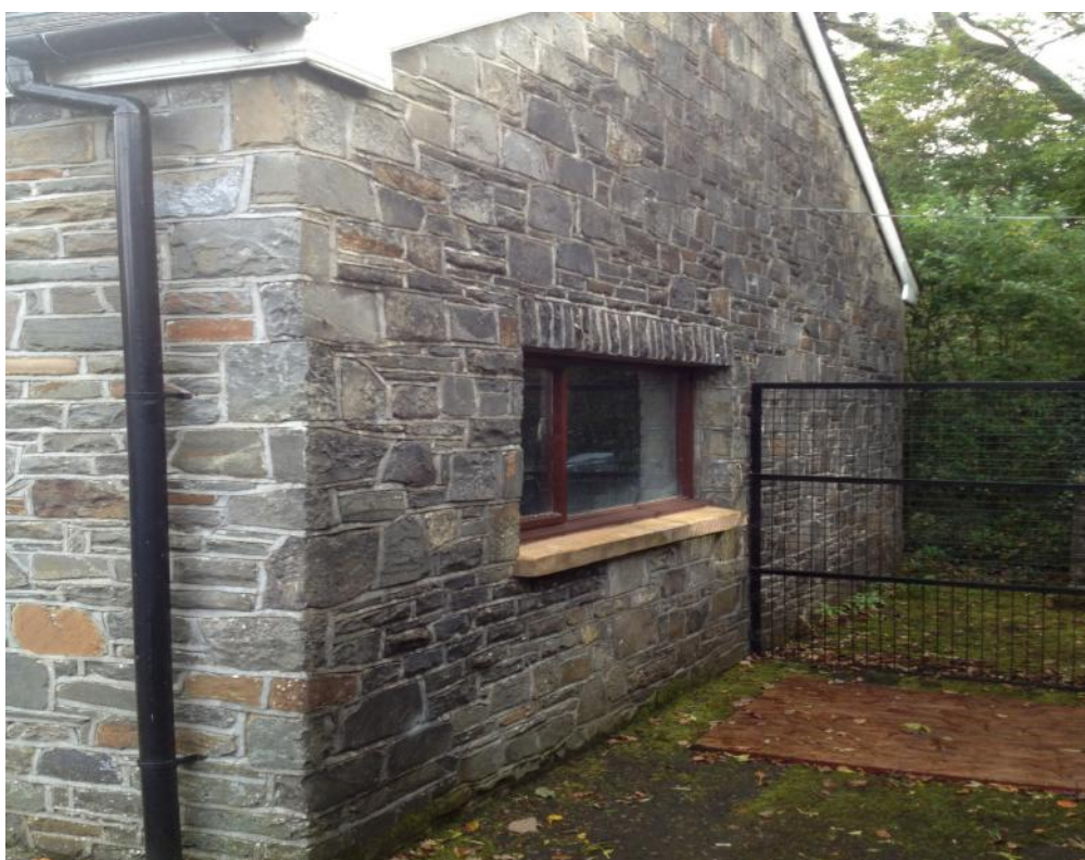
Existing south facing elevation of barn number 1.
