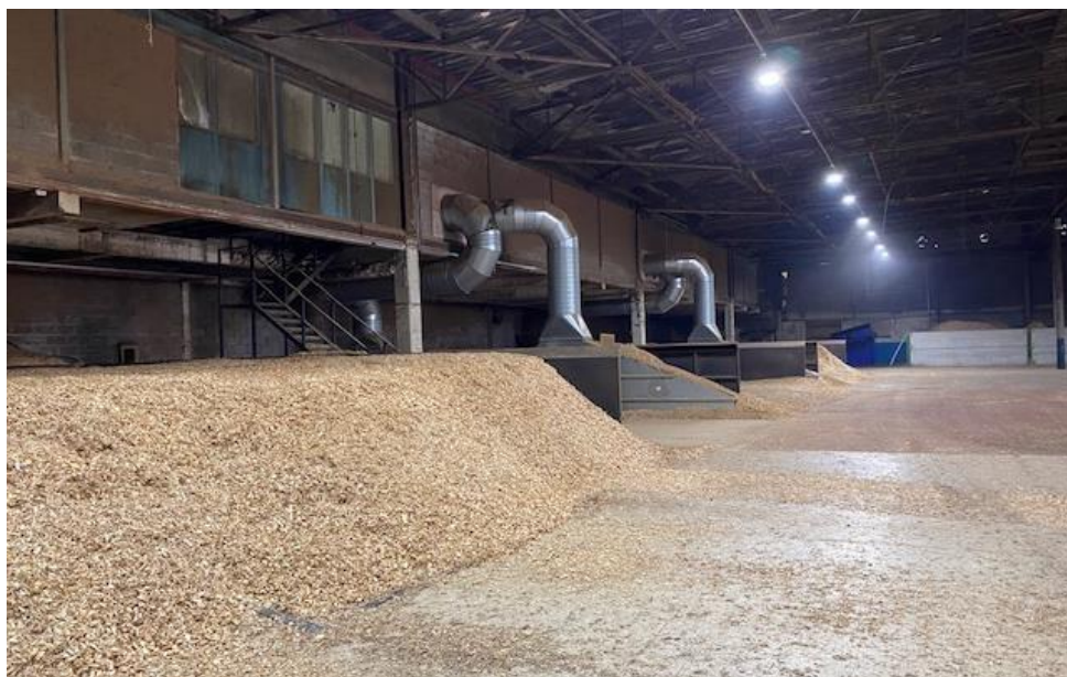
Photo 1 – existing internal storage of woodchip with drying beds on show
