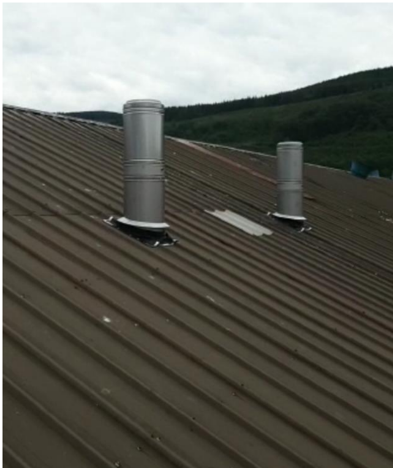
Photo 5 – existing roof-top external flues at Vale of Neath Business Park
