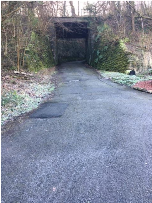
Photo 1 - View from the site access looking East towards the viaduct.
