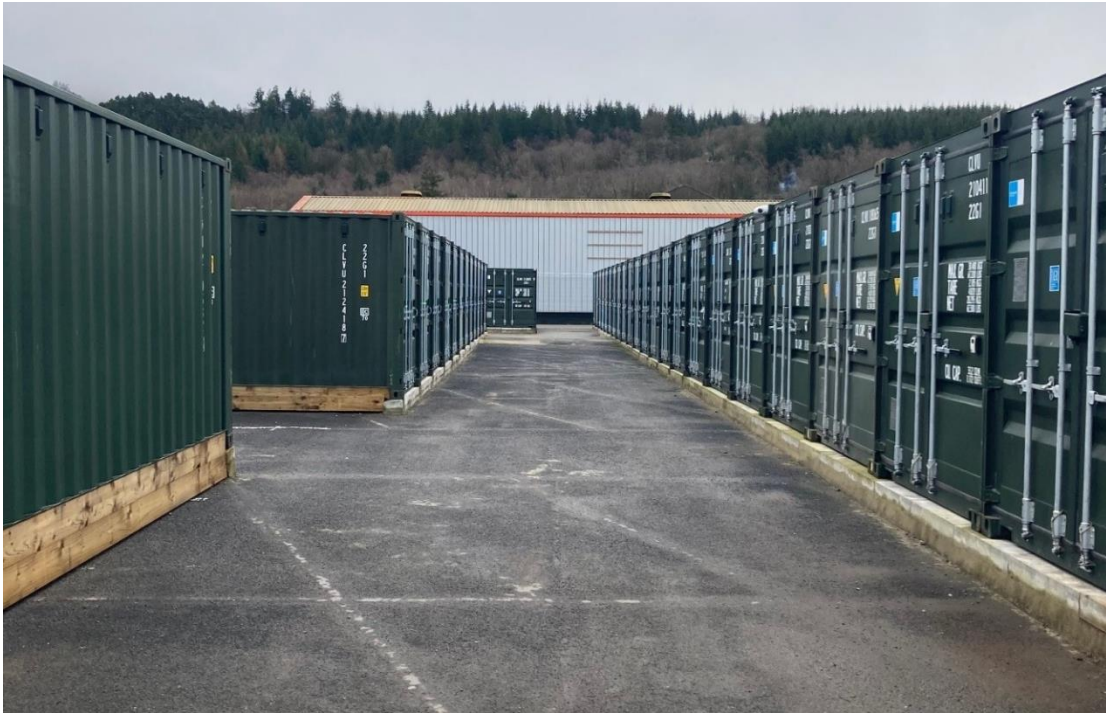
Figure 2-4 Steel container based self-storage facilities at the site
