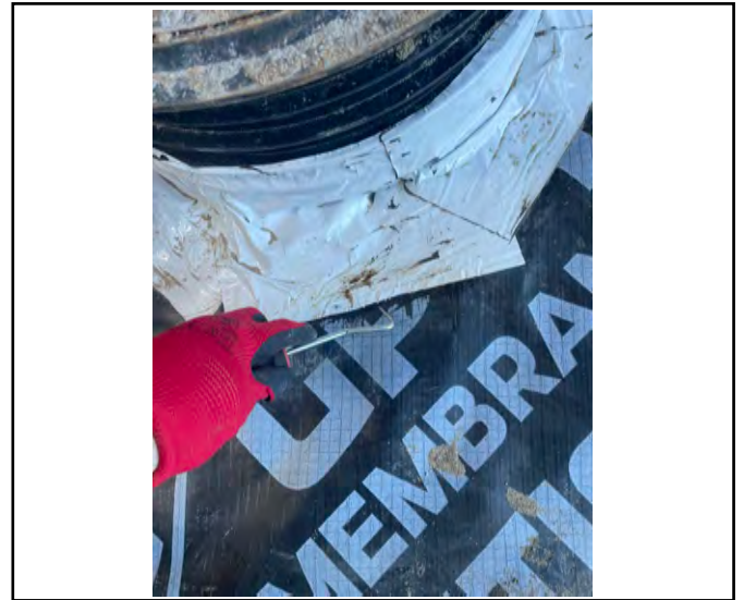
Pick and probe test carried out to a sealed man hole.
