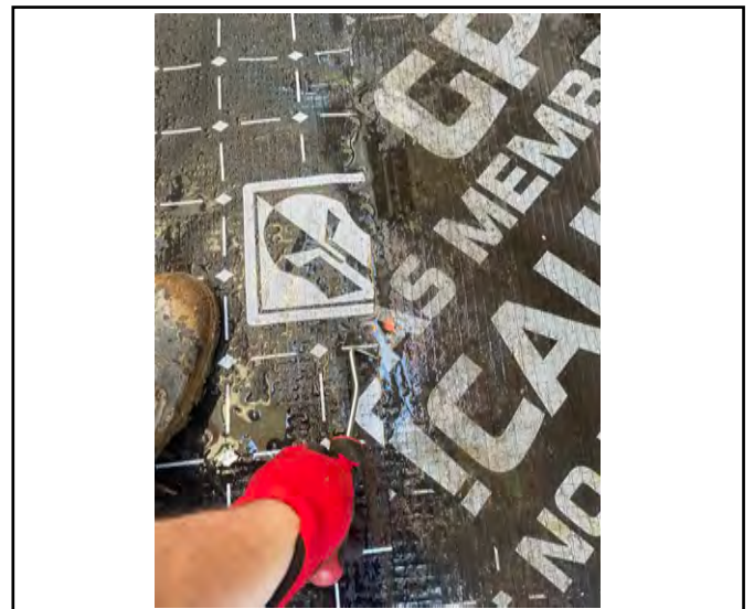
Additional pick and probe test carried to a welded lap of the membrane.
