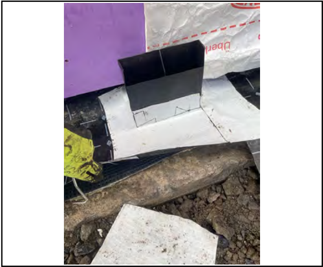
Identifying pressure relief vent mat.
