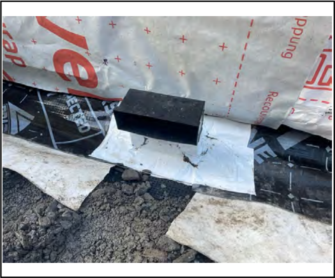
Successfully sealed periscope vent.
