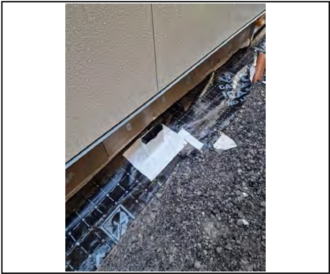
Successfully sealed periscope vent.
