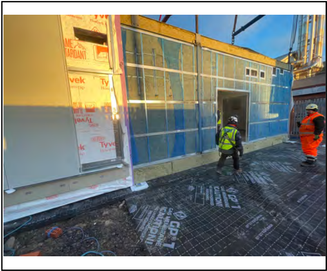
Module dropped into place, no damage caused.
