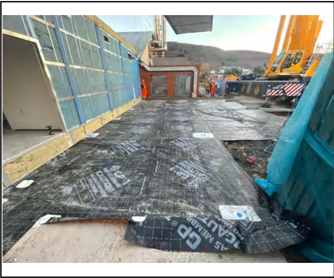
Overview of gas barrier before module was dropped into place.
