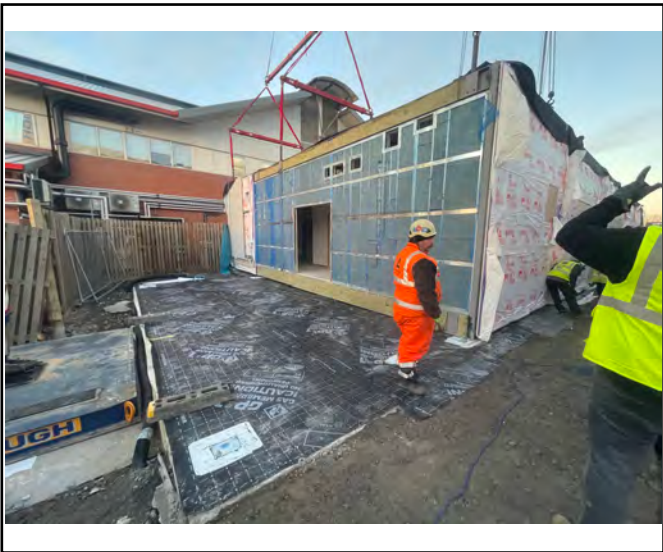
Module dropped into place.
