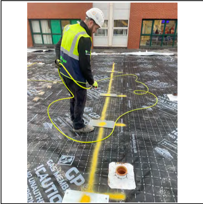
Air lance test to welded lap.
