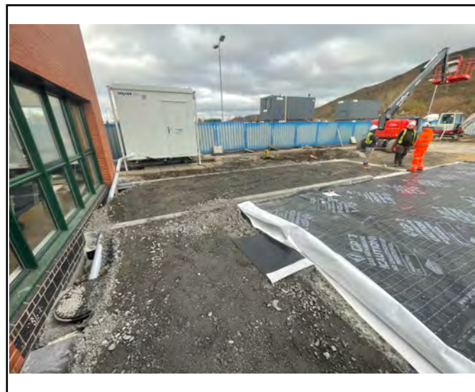
Additional overview of one of the bays to be sealed.
