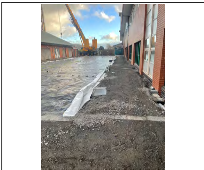
Overview photograph of area where three bays are still to be installed.
