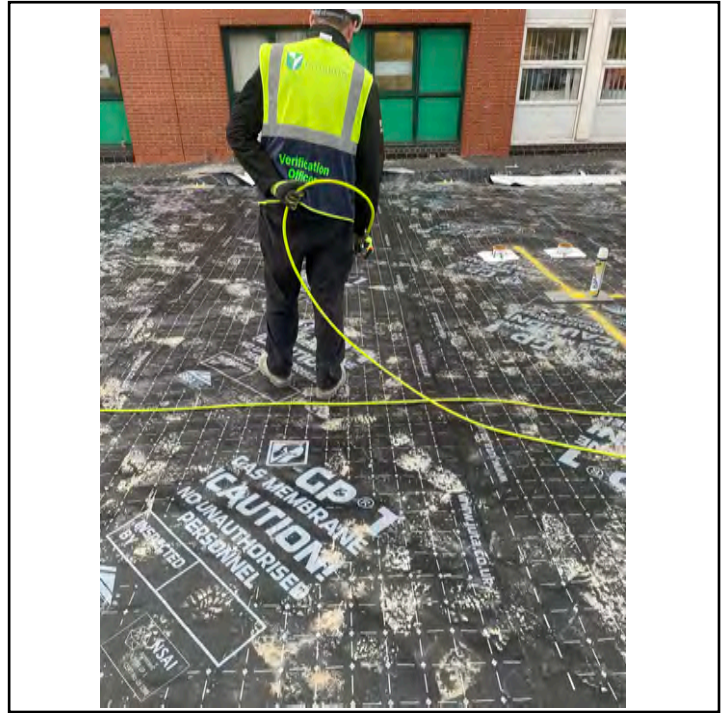
Air lance test to welded lap.
