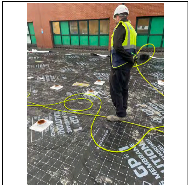
Air lance test to sealed pipe penetration.
