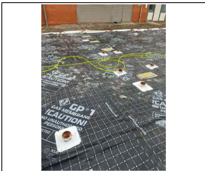
Additional sealed details using JUTA
