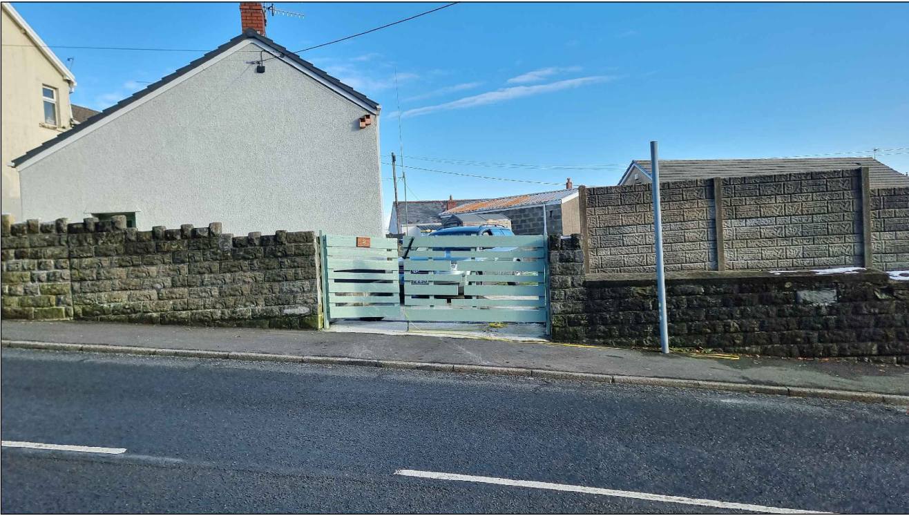
EXISTING ACCESS & GATES SUBJECT OF APPLICATION
