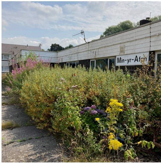
Figure 4. Single storey building with a flat roof.
