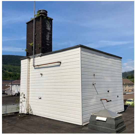
Figure 5. Additional structure on the roof to the east.
