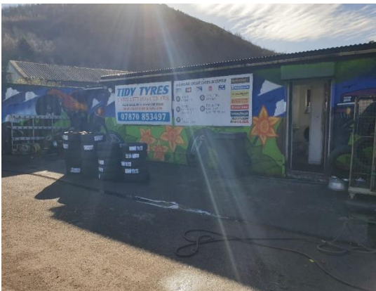
Offices, Toilets and Storage
