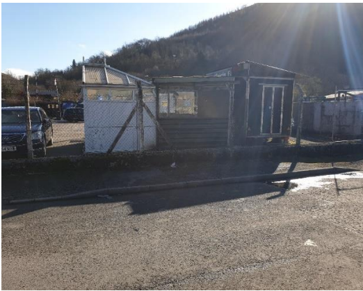
Street view of Sheltered Seating
