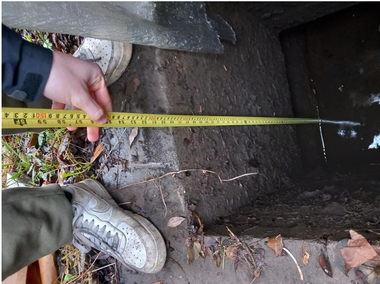
Storm water run-off discharged into natural water course Swansea canal.
