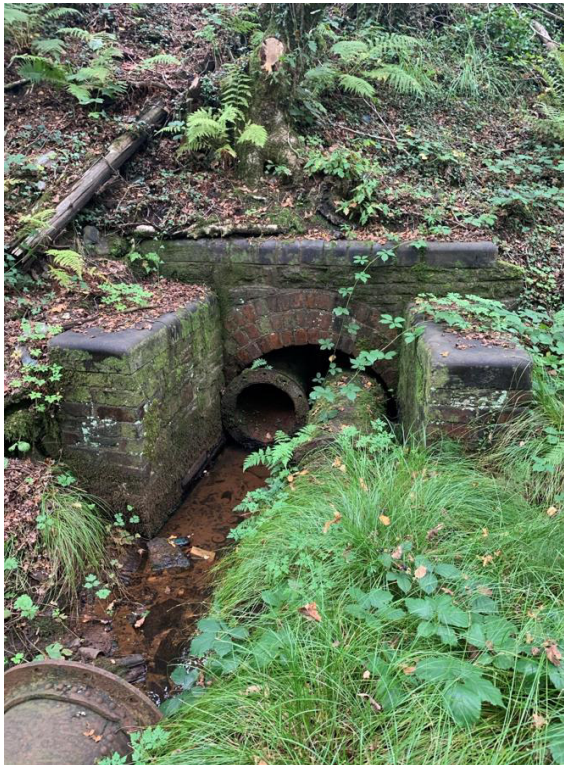
Figure 5: Network Rail 1.5m diameter Culvert & Watercourse looking East
