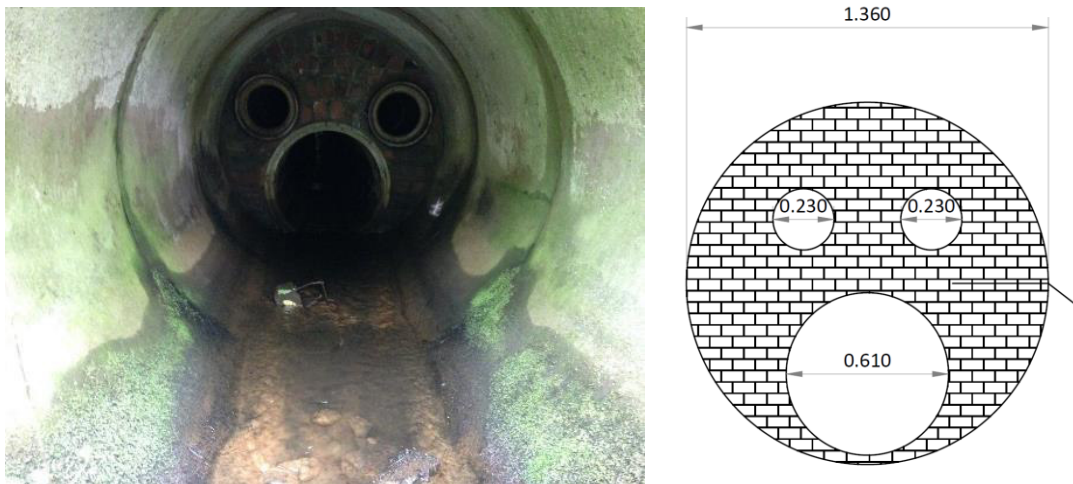
Figure 7: Culvert & Internal Pipe Arrangement Under Private Railway Siding looking West
