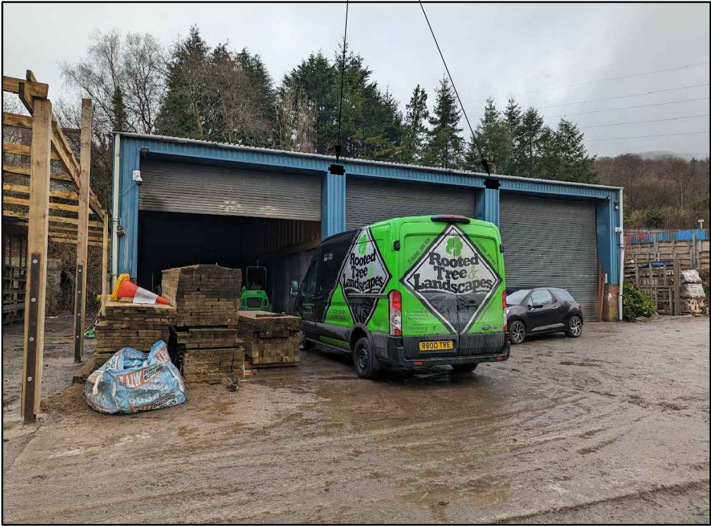
Photograph showing the existing building
