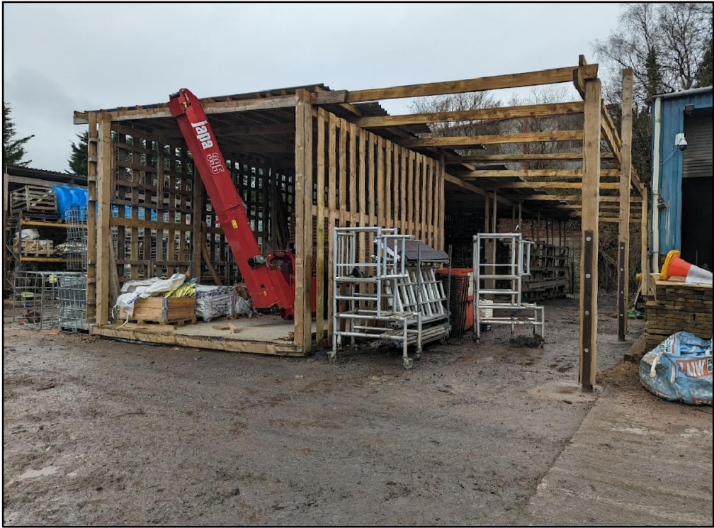
Photograph showing the extension to shed 1. The purpose is to provide workers with a sheltered area to work in
