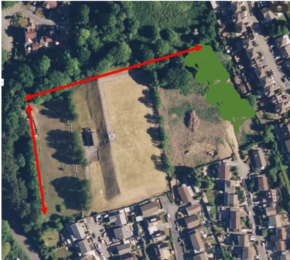
Aerial site image (courtesy of Apple maps™)
