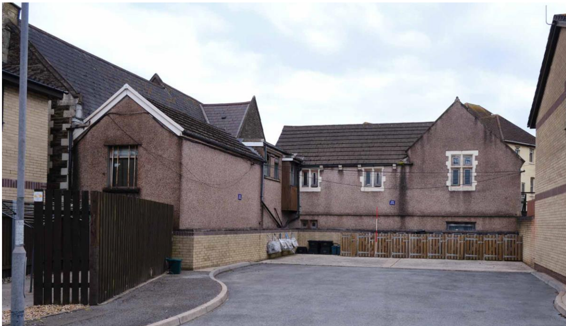
Figure 8. South-east (rear) front facing Eagle Mews.
