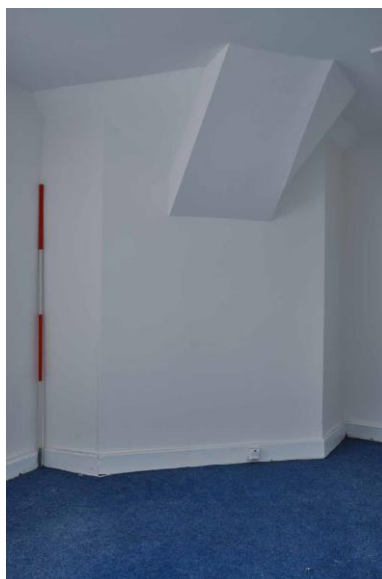
Figure 10. Position of first-floor fireplace in front range.
