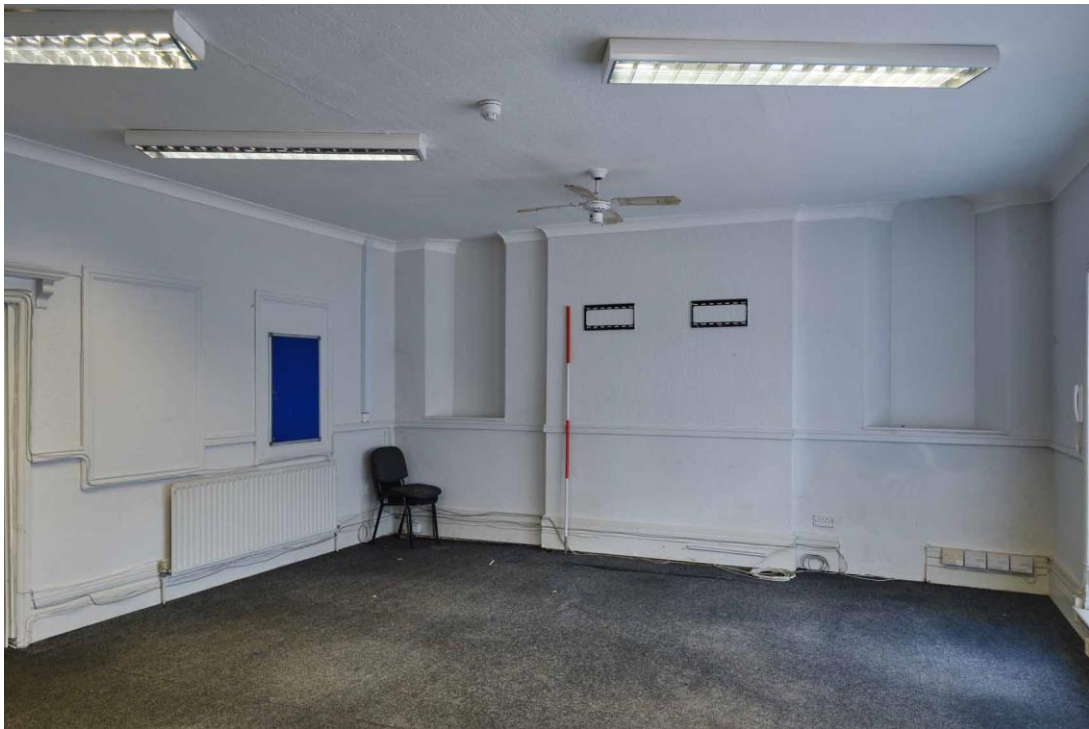
Figure 9. Blocked windows and fireplace in the ground floor of the front range.
