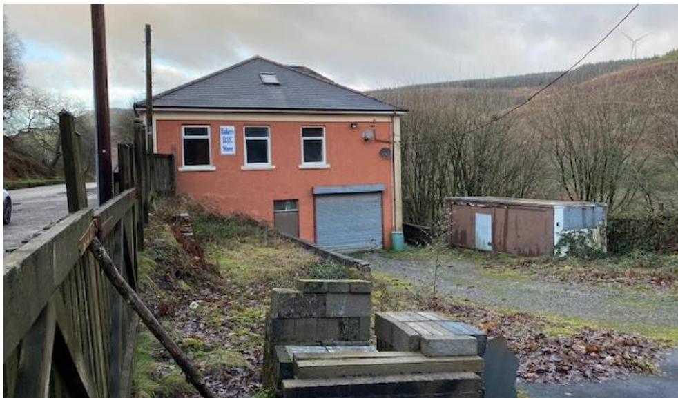
Photo 2 – view of eastern side of building and its lower ground floor to rear from adjoining parking yard
