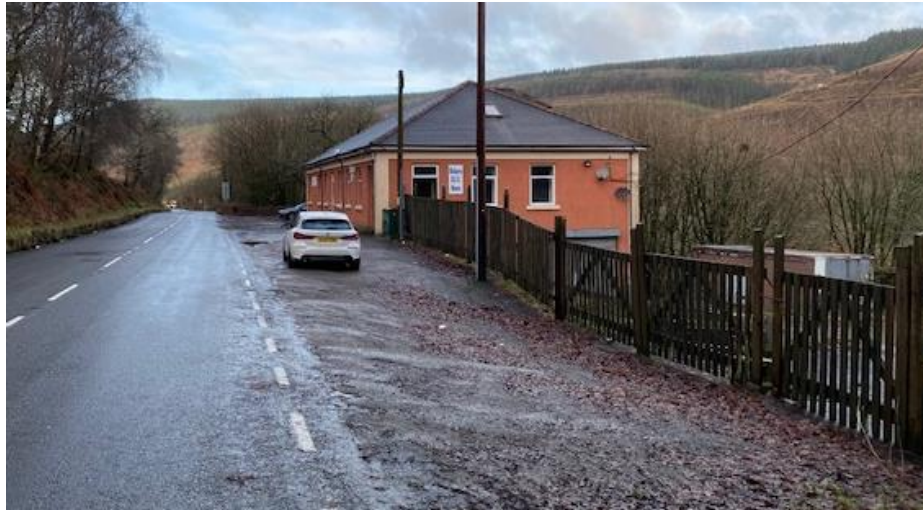
Photo 3 – view looking west along road frontage and extent of wide front hardstanding
