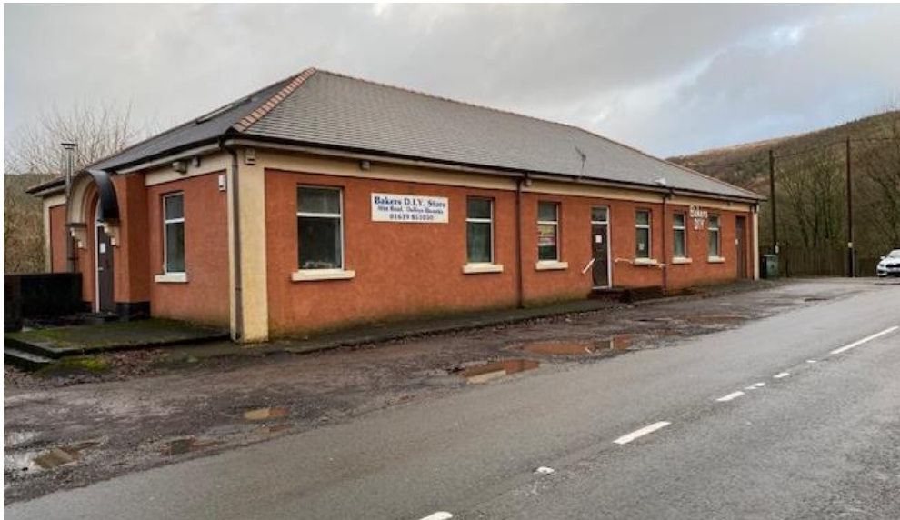
Photo 1 – existing workshops viewed from Afan Road carriageway
