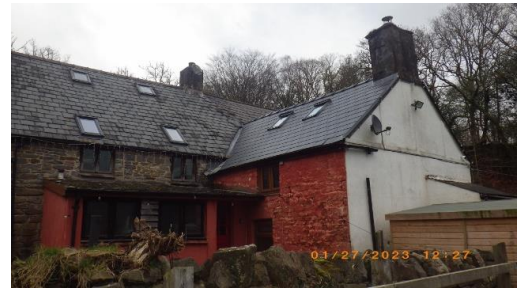
West elevation of the house and the adjoining property.
