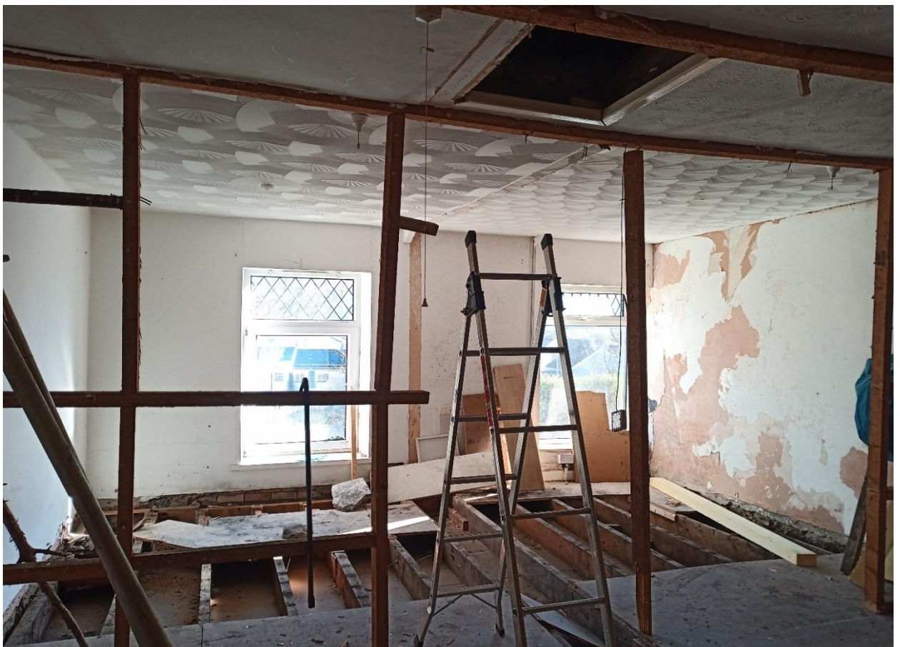
Figure 4: First floor interior facing eastward
