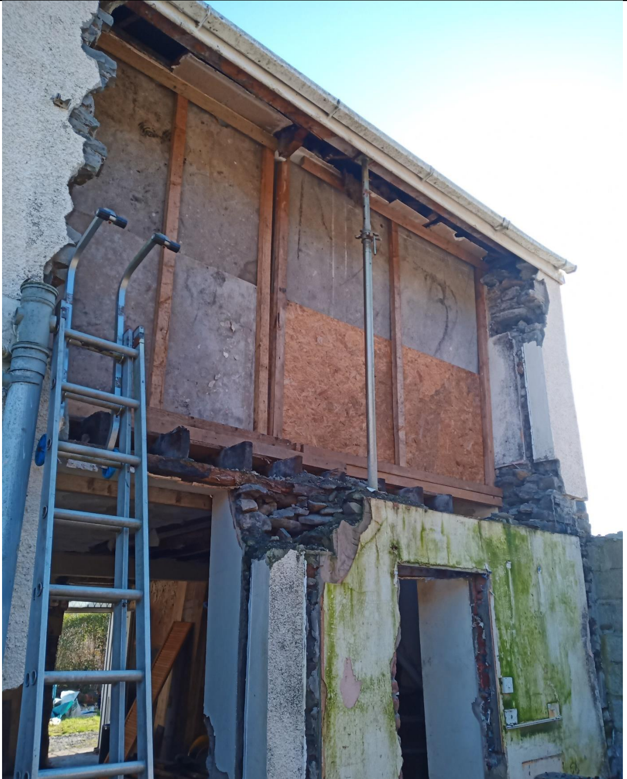
Figure 2: West elevation from the ground floor showing boards and exposed stonework
