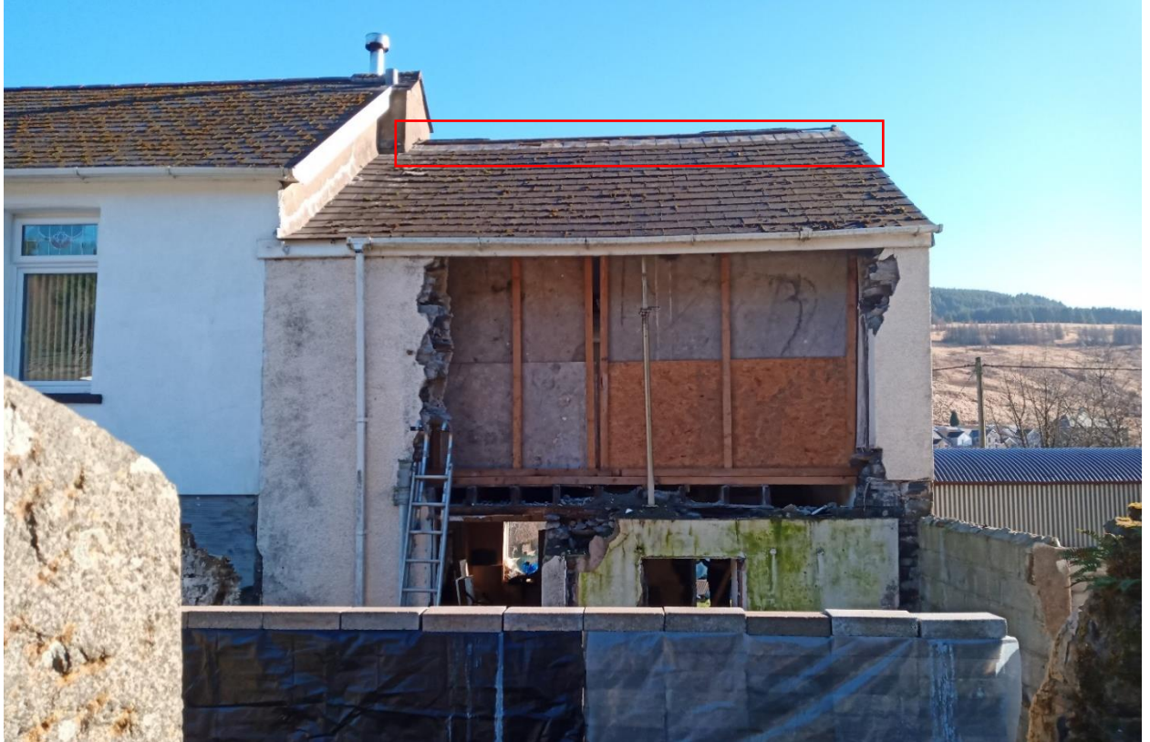
Figure 3: West elevation showing the removed ridge tiles highlighted in red
