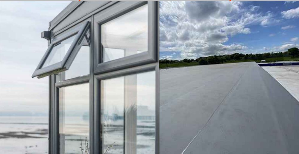
Anthracite UPVC Windows Upper Floors Residential Units
