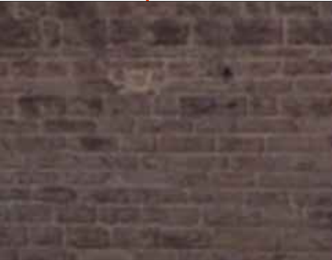
Reclaimed Stone to Boundary Wall
