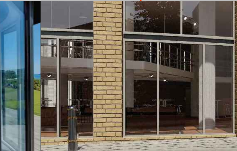
Anthracite Powder Coated Aluminium Windows & Doors to Ground Floor Commercial Units
