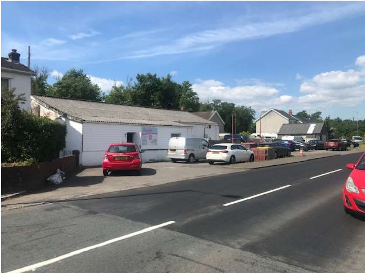
Exterior view of the site looking north
