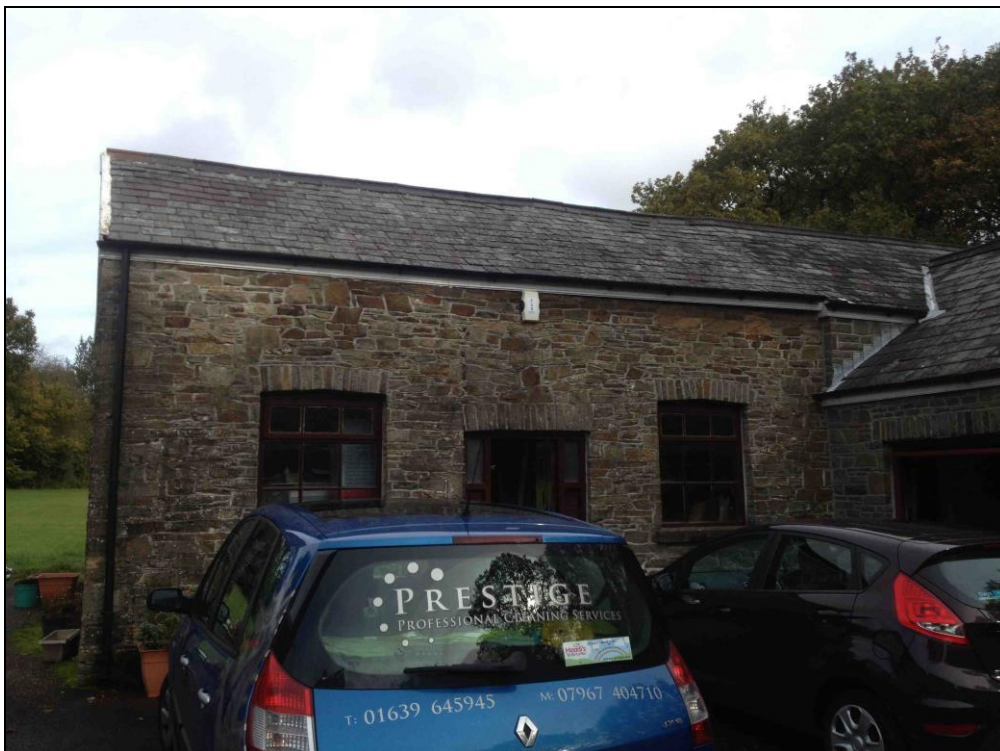
Photo 3: Original western extent of northern stone barn (view looking north).
