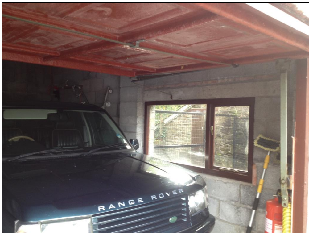
Photo 6: Interior of modern eastern garage.
