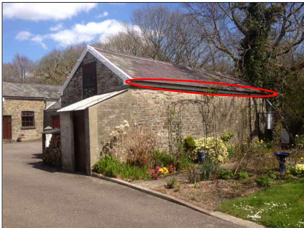
Photo 9: Approximate location of roosting Soprano Pipistrelle beneath wooden fascia on southern elevation of southern barn.
