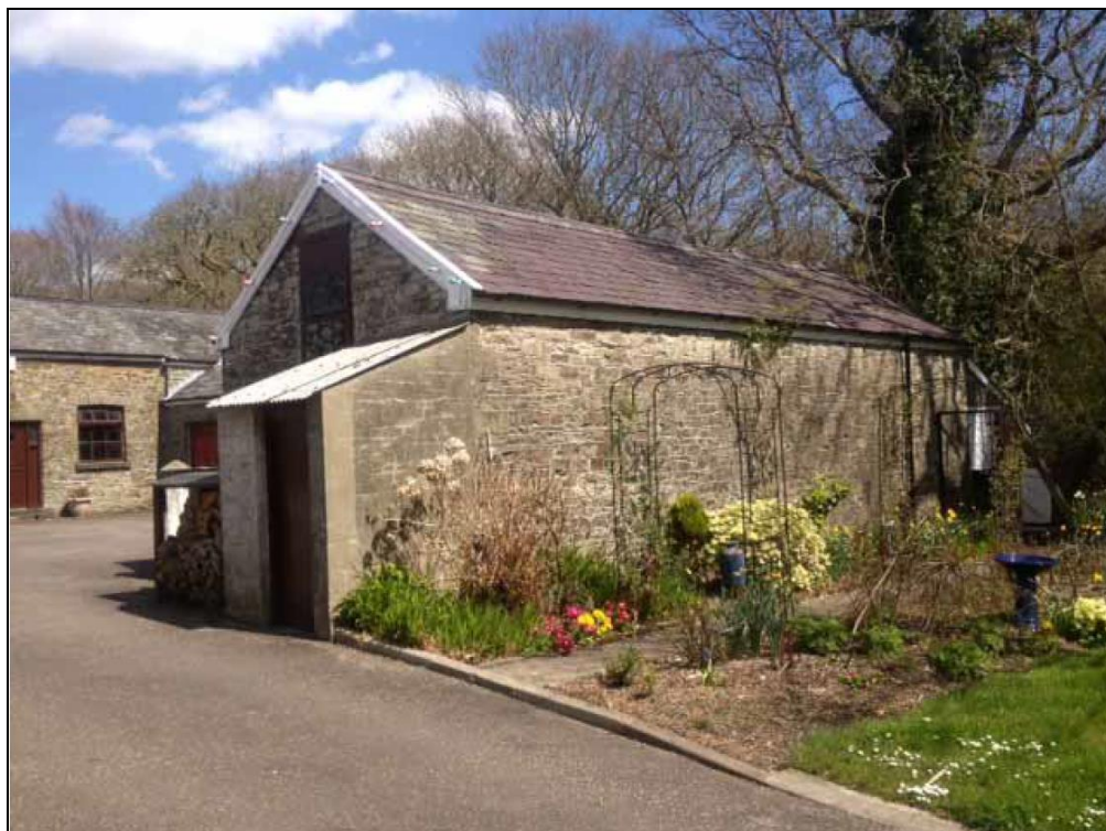
Photo 2: Western gable end and southern elevation of southern barn (view looking north).
