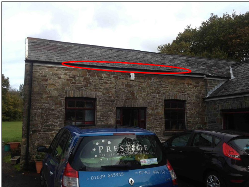
Photo 8: Approximate location of roosting Pipistrelle on southern elevation of northern barn (view looking north).
