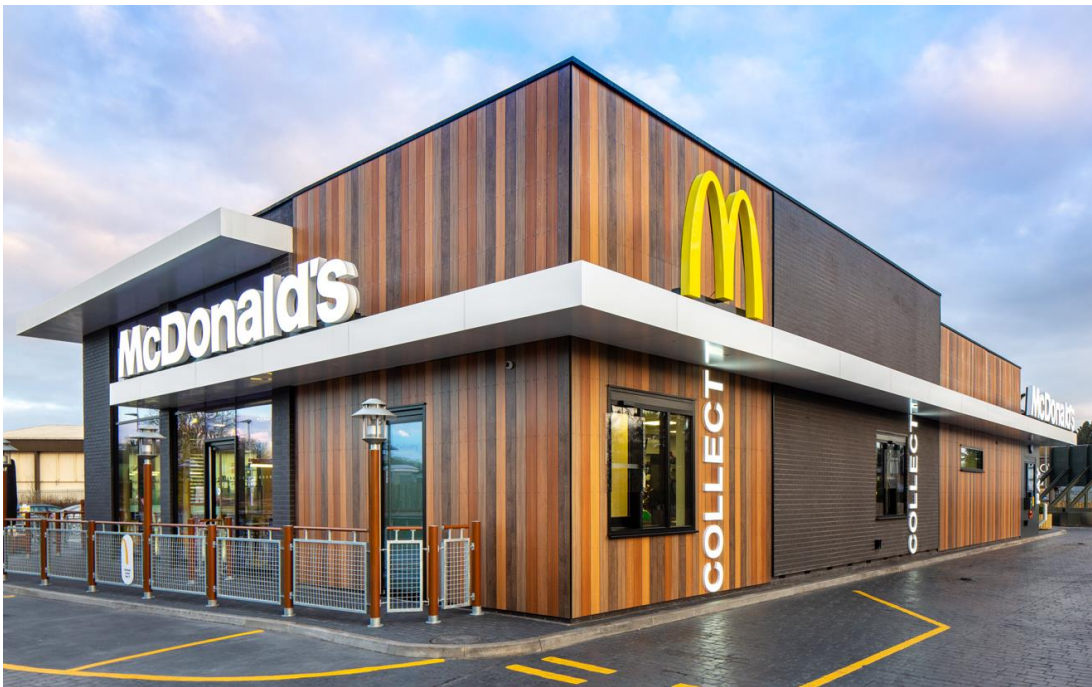
Example of the building
