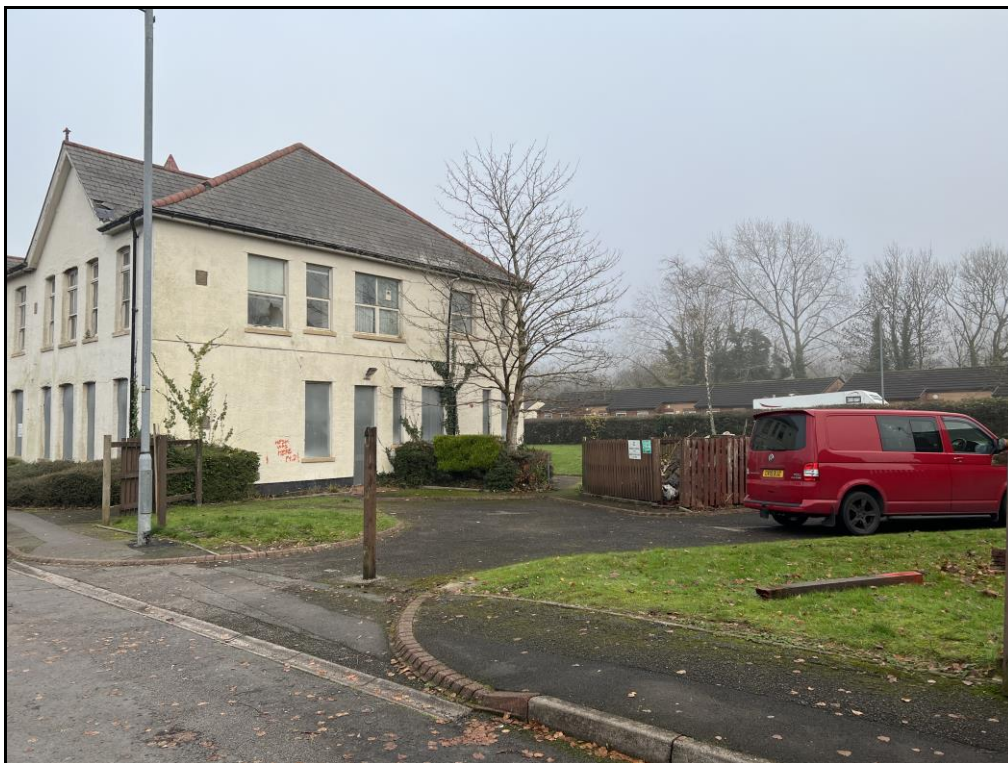
Plate 2: View northeast towards the southwest face of the existing building showing trees and hedge line.
