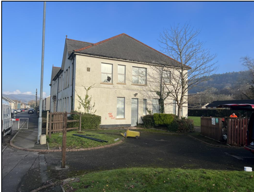
Plate 1: View northeast towards the southwest face of the existing building at area of proposed development footprint.
