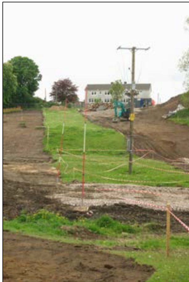
Plate 20: Area J before topsoiling from the east
