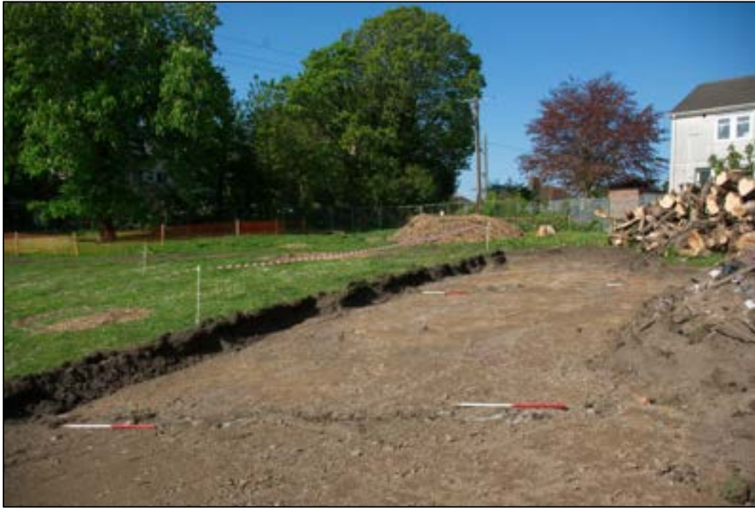
Plate 15: Area F, drains (17) and (19) from the east
