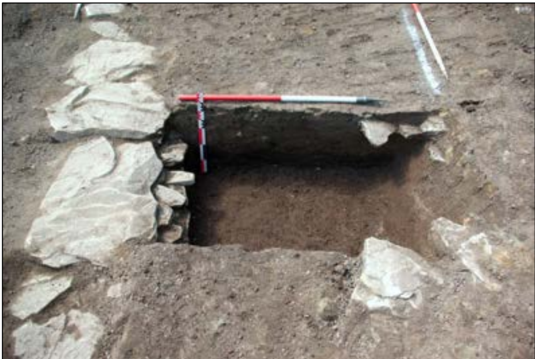
Plate 14: Area F, wall 23, section 02 from the north
