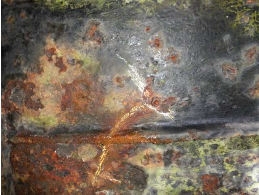
Photo 14: Diagonal Fracture to Upside Panel (07.08.21)
