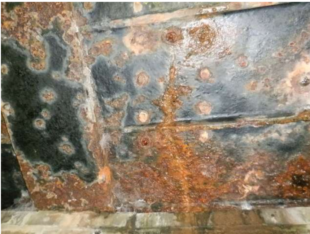
Photo 13: O/S Transverse Fracture to Upside End Panel (07.08.21)
