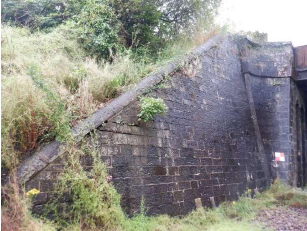
Photo 30: Downside Low Mileage Wingwall (07.08.21)
