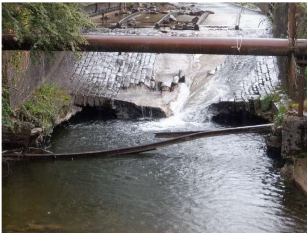
Photo 37: View of Weir (07.08.21)
