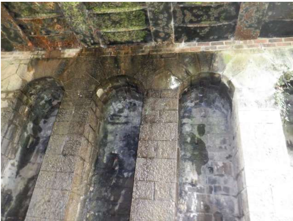
Photo 29: Water Flow Between 2nd & 3rd Relieving Arch (07.08.21)
