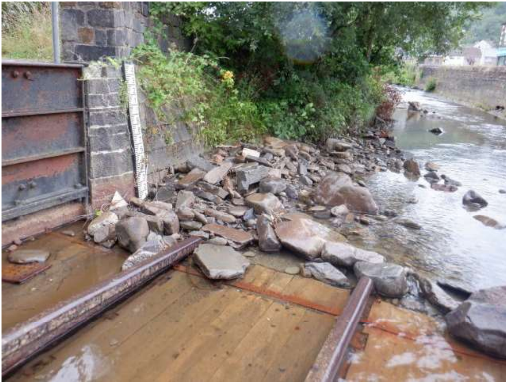
Photo 15: Large Stones Resting on Sacrificial Timbers (07.08.21)
