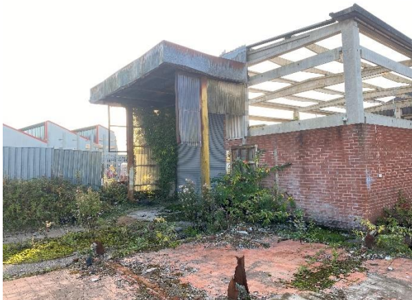
Photo B3-GA1 – Front entrance elevation on gridline 1
