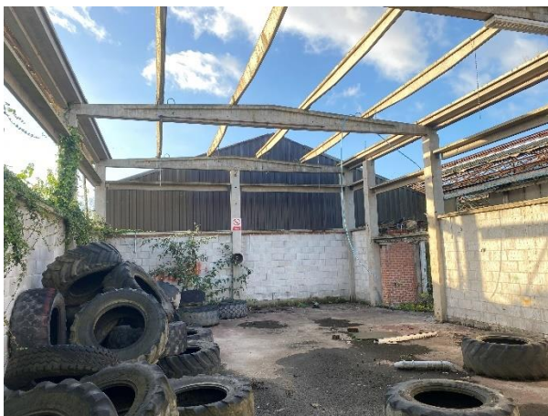
Photo B3-GA5 – Internal elevation on gridline 4
