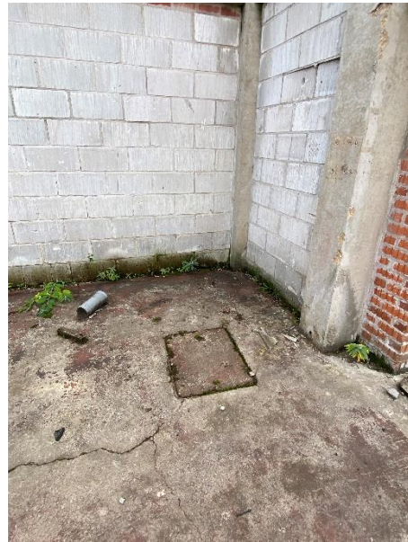
Photo B3-GA10 – Internal manhole
