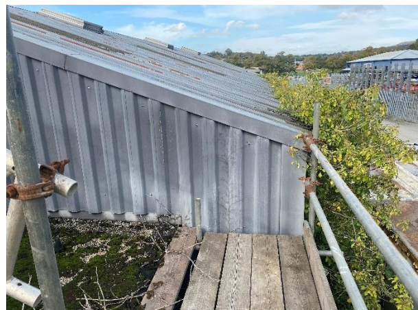
Photo B2-GA4 – External roof along gridline I
