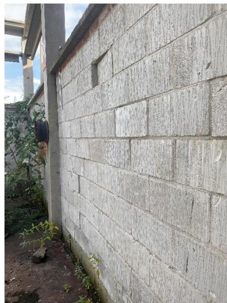
Photo B3- D4 – Further impact damage to masonry panel on GL 4
