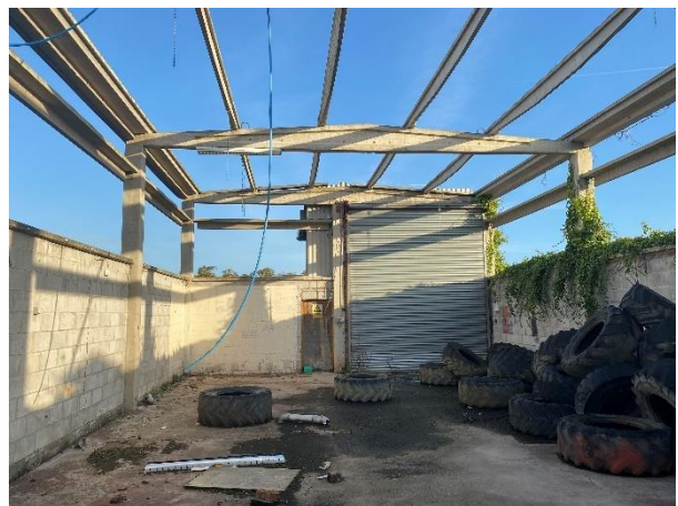
Photo B3-GA6 – Internal elevation on gridline 1
