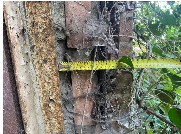
Photo B2- D3 – Masonry repairs to emergency exit on gridline I
