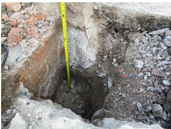
Photo B1 - GA7 - Trial pit to column on gridline A1
