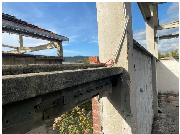
Photo B3-GA8 – Typical cladding rail – note upper concrete rebate/lip for connection of cladding J bolt fixing
