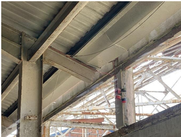
Photo B2-GA7 – Valley gutter along gridline F
