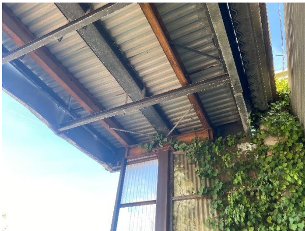
Photo B3-GA11 – Underside of canopy on gridline L
