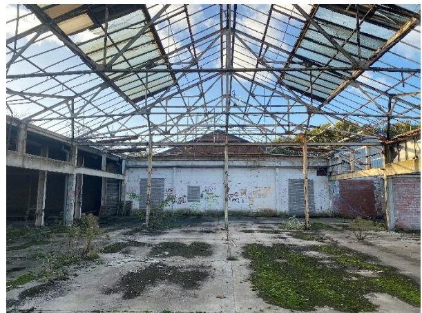
Photo B1 - GA6 - Internal elevation on gridline 10
