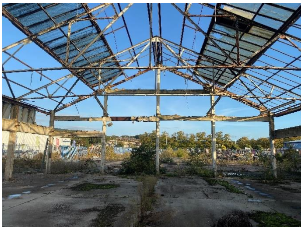
Photo B1 - GA5 - Internal elevation on gridline 1
