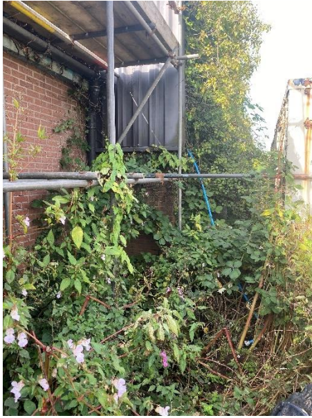
Photo B2-GA5 – External building corner on gridline I/11
