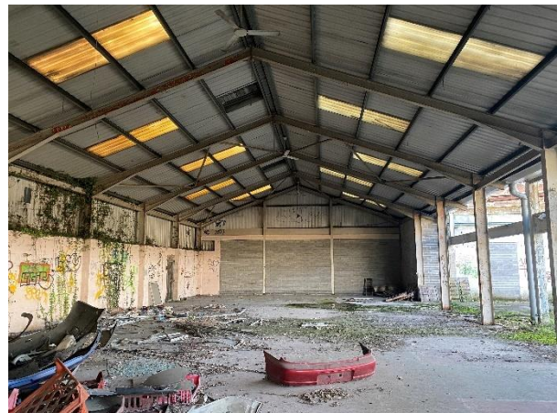
Photo B2-GA2 – Internal elevation on GL11
