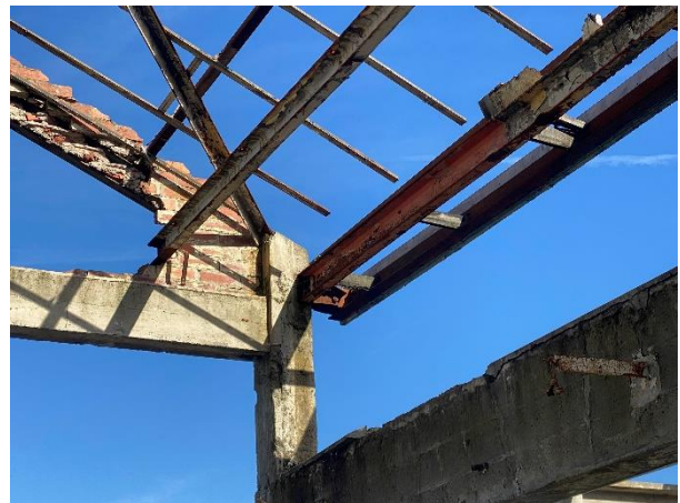
Photo B1- D8- Twisted end to purlin
