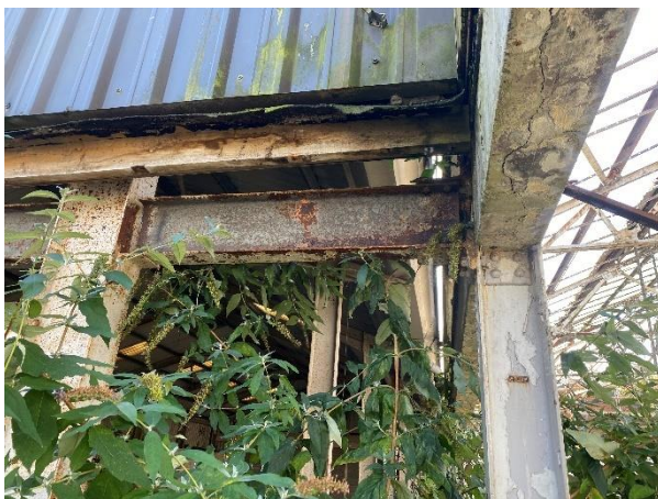
Photo B2-GA9 – Building 1 to building 2 connection on gridline F4
