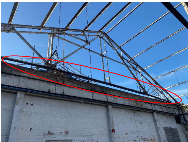
Photo B1- D1 – Bracing required
