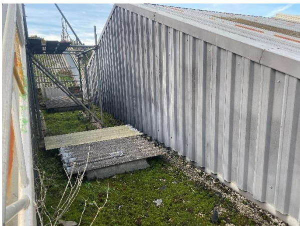
Photo B2-GA3 – External elevation on GL11
