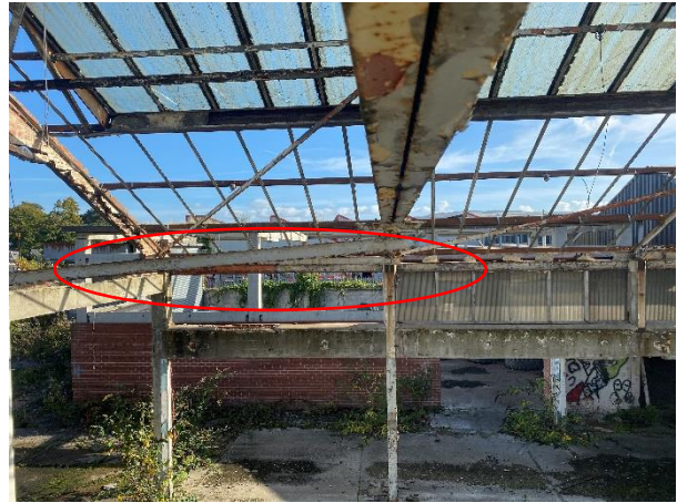
Photo B1- D10- Redundant steel beams to be removed circled in red
