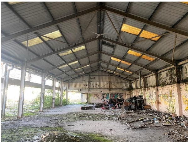
Photo B2-GA1 – Internal elevation on GL4
