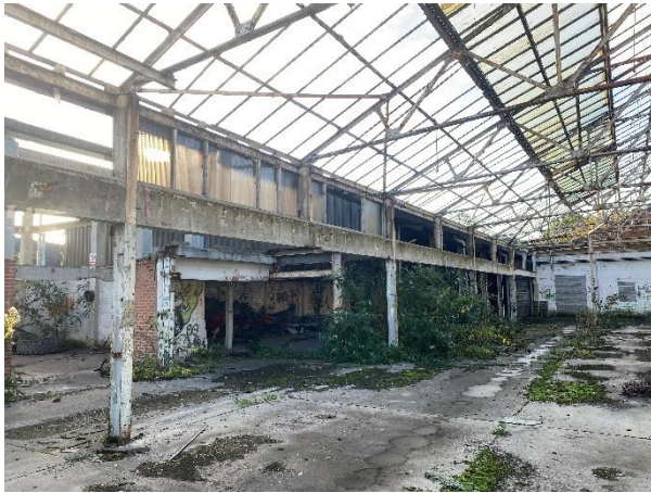
Photo B1 - GA3 - Internal elevation on gridline E
