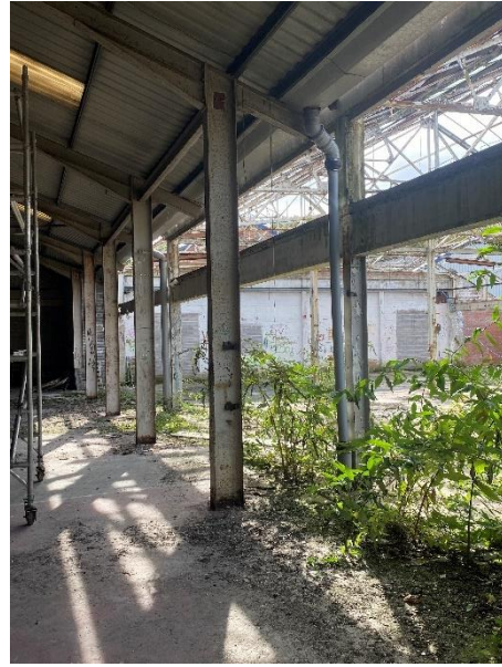
Photo B2-GA6 – Building 1 to building 2 joint arrangements
