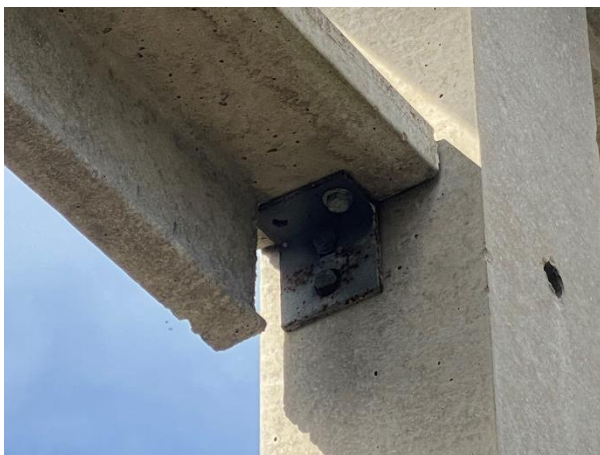
Photo B3-GA7 – Typical cladding rail to column connection
